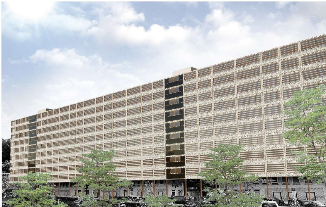
Figure 64a, façade system integrated in the building in Amsterdam, SIDE 4.
