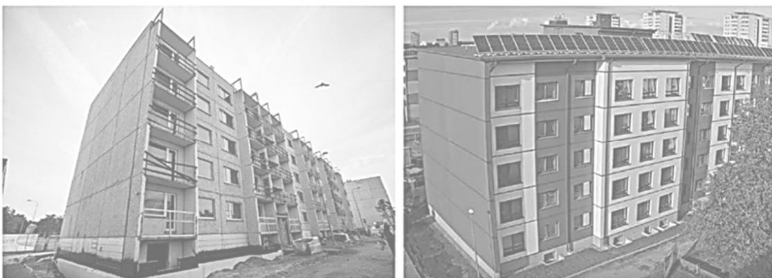
Figure 27. Before (left) and after (right) the renovation source: (More-Connect 2019)
