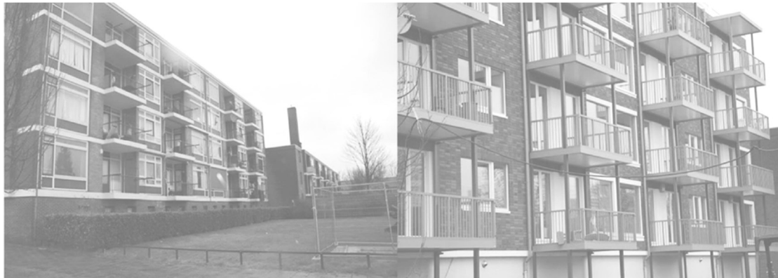
Figure 25, Before (left) and after (right) the renovation source: (More-Connect 2019)
