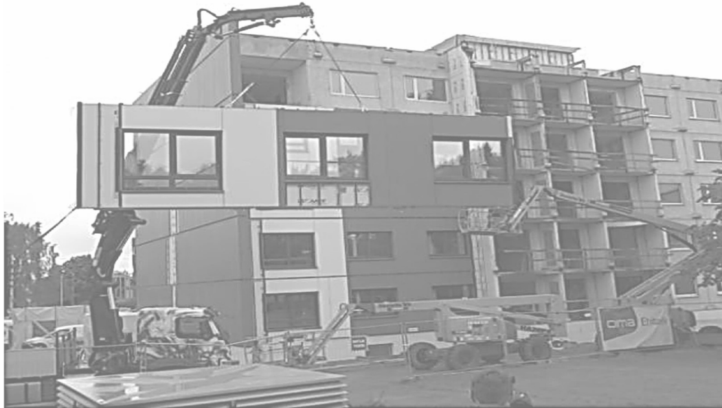
Figure 26. Installation of the module panels on the walls source: (More-Connect 2019)
