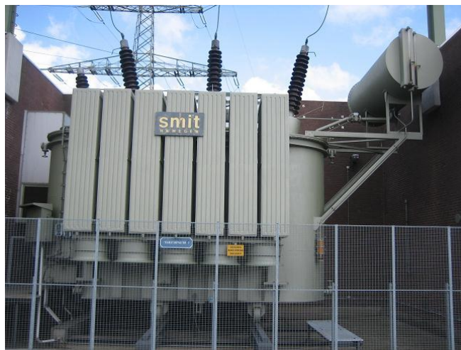
Fig 2.4: Example of a HV/MV transformer designed by SMIT
