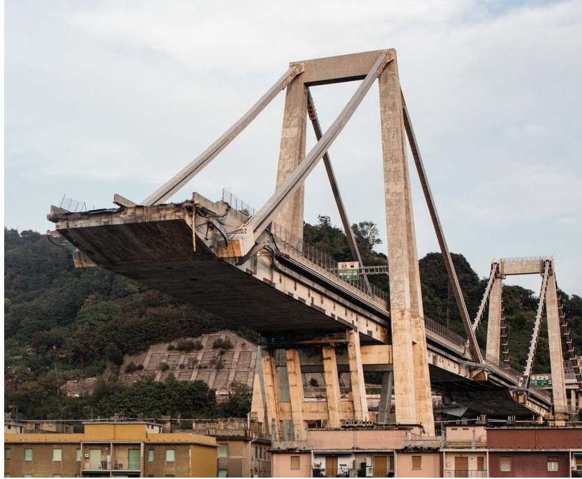
Figure 1.1: Collapsed Morandi bridge, Genua, Italy [19]
