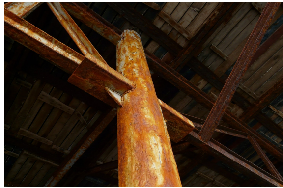
(b) Corrosion of steel elements (pixabay, n.d.)
