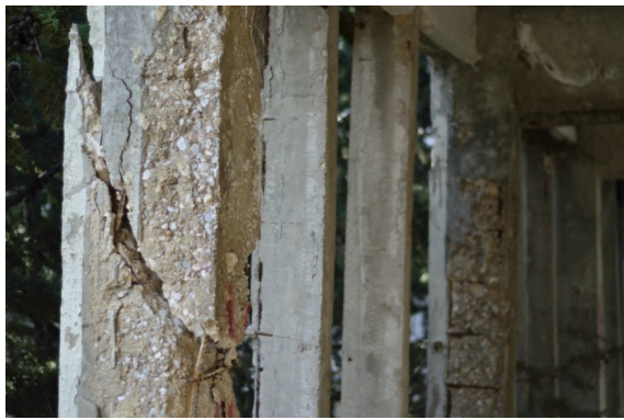
(a) Deteriorating reinforced concrete elements (Adobe Stock, n.d.)
