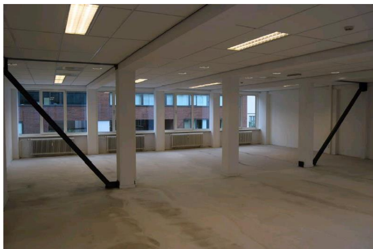
Figure B.9: Bracings in the existing building of de Gekroonde P (Ventu, 2020)
