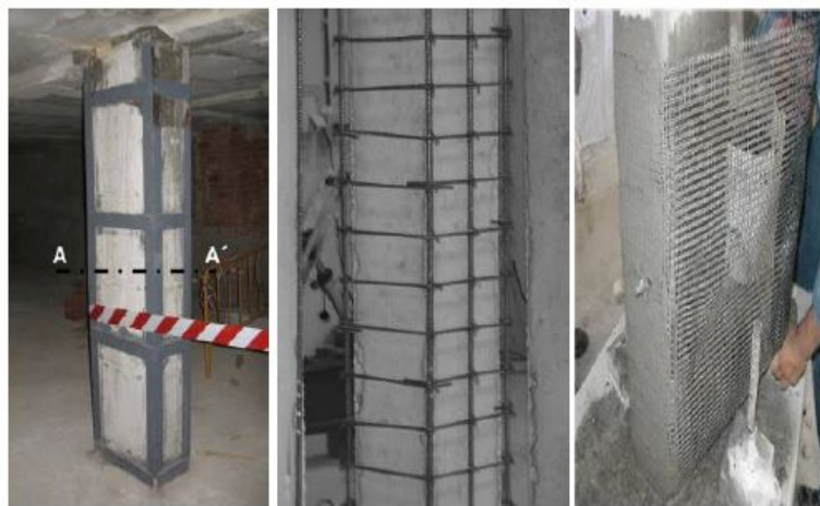
Figure 2.17: Column strengthening: steel jacketing, concrete jacketing, FRP jacketing (Islam and Hoque, 2015)
