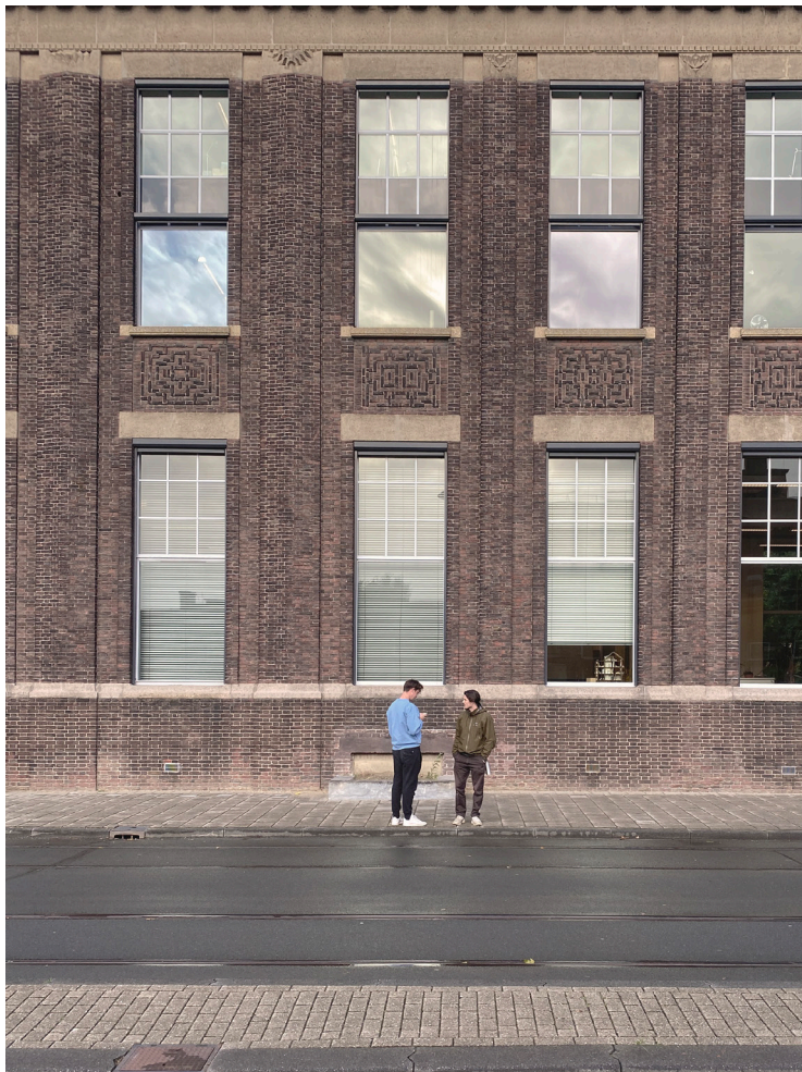
Non-utilized building front
