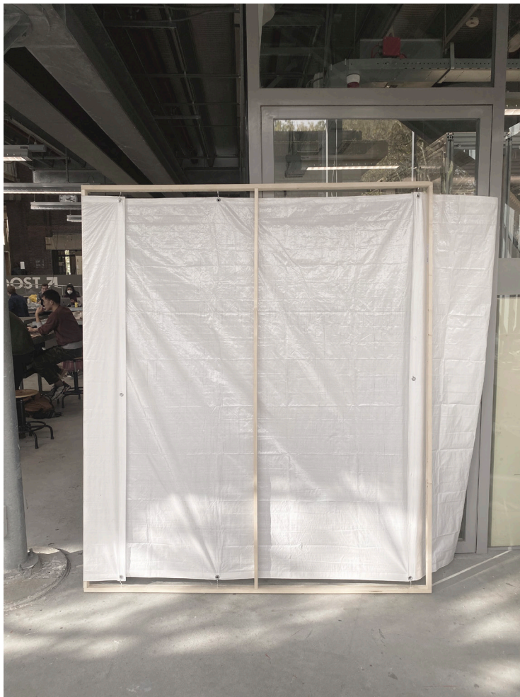
Construction of the awning
