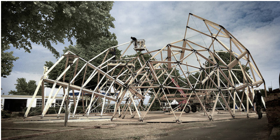
Fig. 7.7 - A lattice structure made of wood connected with steel nodes [Source: http://www.archdaily.com/276056/peoples-meeting-dome-kristoffer-tejlgaard-benny-jepsen ]
