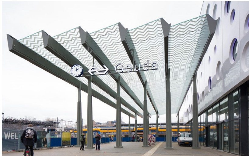
Fig. 5.14 - The stiffening glass elements to stabilize the steel construction on the station of Gouda. [Haarhuis et al., 2016]
