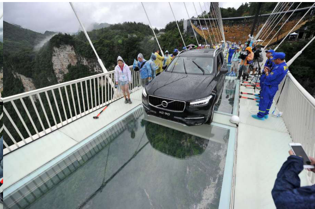
Fig. 4.18 - Driving a car over the bridge to demonstrate the safety of the structural glass. [Source: https://www.thestar.com/news/world/2016/08/03/china-opens-terrifying-tianmen-mountain-glass-walkway.html ]
