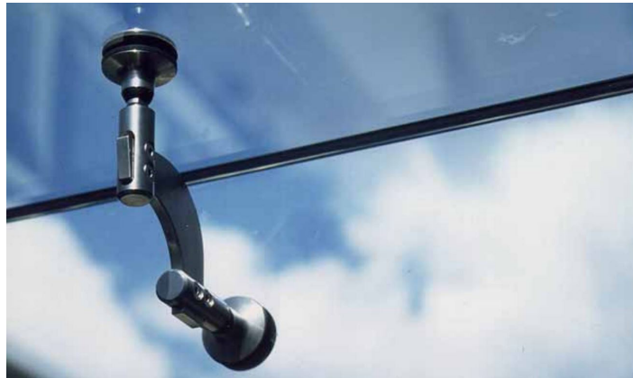
Fig. 4.24 - Point fixed detail of the connection between the roof panel and side panel [Kraaijvanger, 1998]
