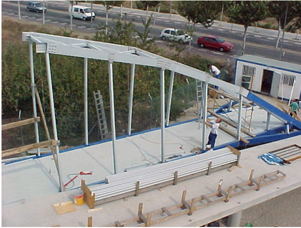
Fig. 4.14 - One half of the arches being painted and constructed. [Source: fiberline.dk]
