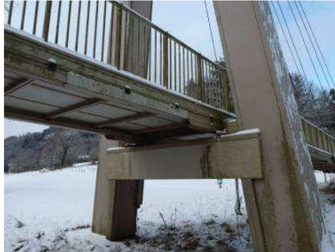
Fig. 4.11 - Close-up of the deck and pylon of the Aberfeldy bridge. [Source: http://compositesandarchitecture.com/?p=2398 ]
