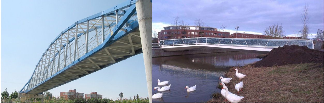
Fig. 1.3 - The development of FRP bridges: from mimicking steel structures to material adapted concepts. [Source: fiberline.dk] [Smits, 2016]
