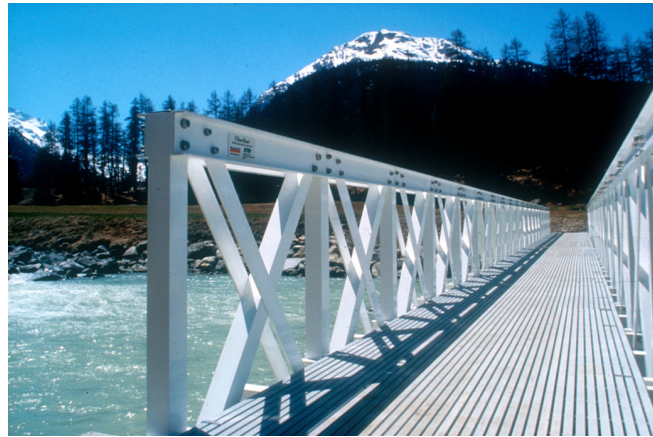
Fig. 4.2 - Close-up on the bolted connections of the trusses of the Pontresina bridge [Keller et al., 2015]
