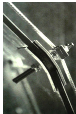
Fig. 3.19 - Contact connection
