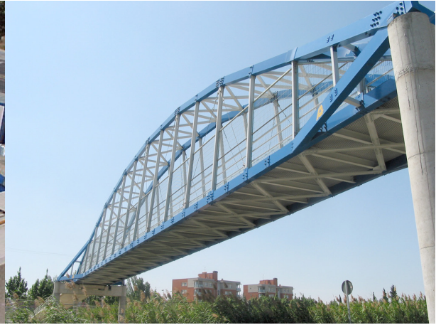
Fig. 4.15 - View on the deck of the Lleida footbridge showing the diagonal and cross beams. [Source: fiberline.dk]
