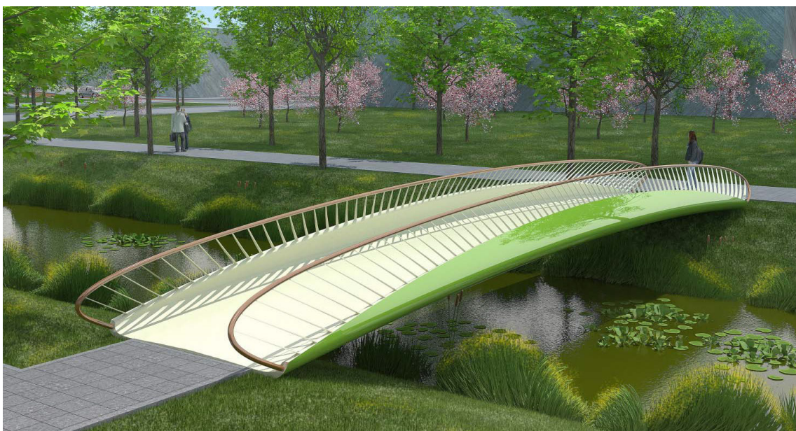
Fig. 2.26 - Shell shaped bridge design: "The cross-section of the deck curves upward, forming part of the bridge's parapet. As the bending momentum increases toward the middle, so does the height of the shell." [Smits, 2016]
