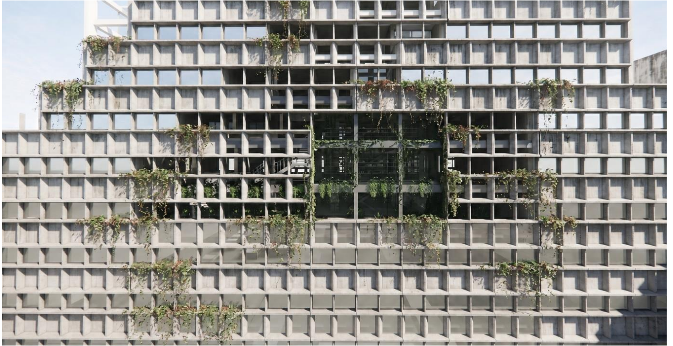
Figure 41: Outside View to the Hybrid Core
