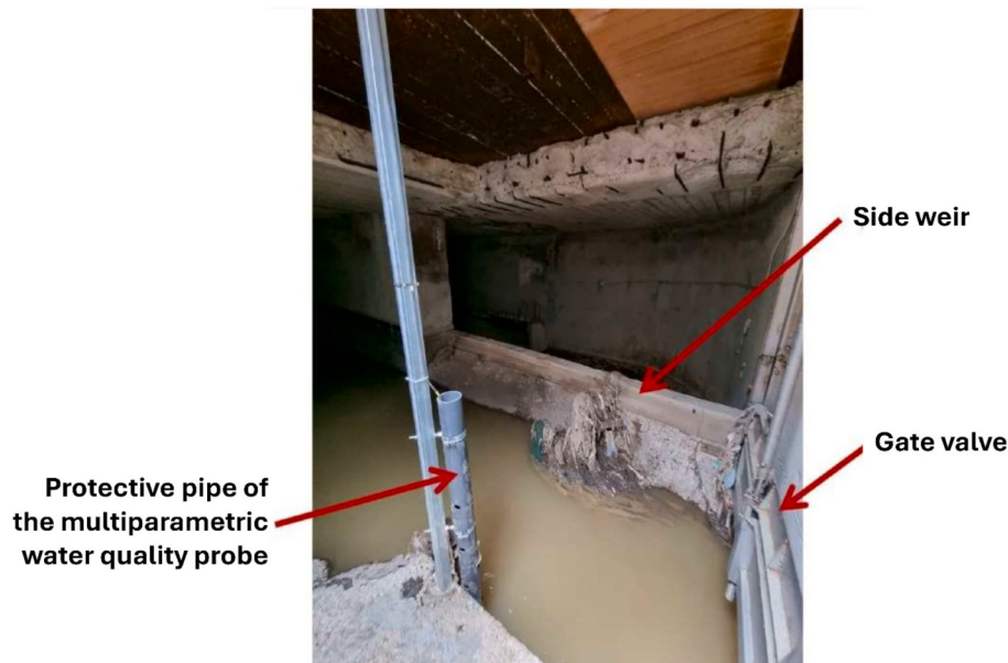
Fig. 4. Overflow structure ( s_2 ), where the water quality multi-parameter probe was installed. The probe was placed inside a pipe to protect it from damage. The side weir, at the centre of the picture; the gate valve, on the right of the picture.
