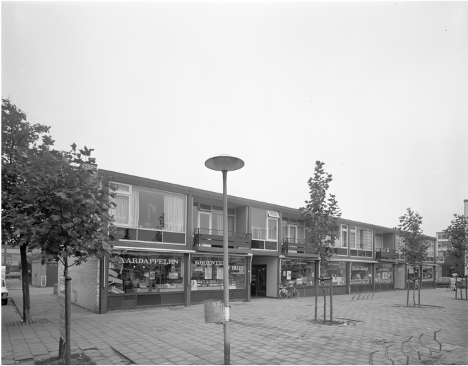
Figure 17. Front facade of two-storey Intervam building before renovation. The window and store front have more transparent appearance than the rear facade.
