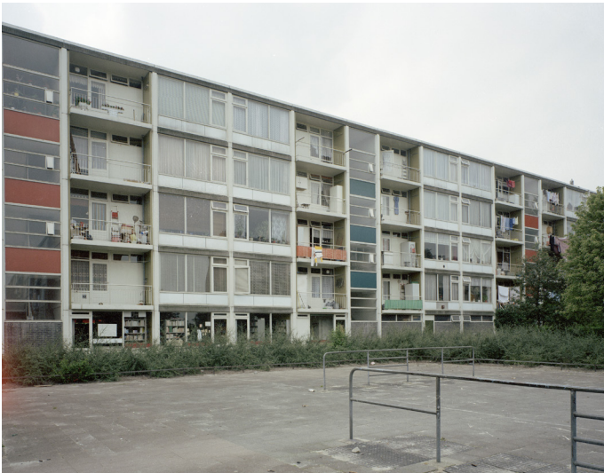
Figure 19. Original facade with wooden window frames
