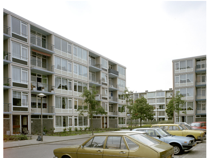
Figure 20. Changed facade with plastic window frames after renovation
