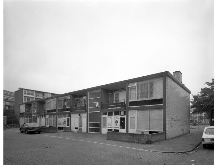
Figure 18. Rear facade of two-storey Intervam building before renovation
