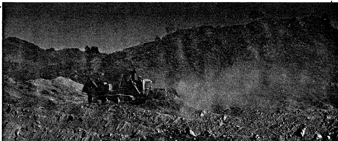
Fig. 22 Catterpillar bulldozer (D9) at work to build a batch.
