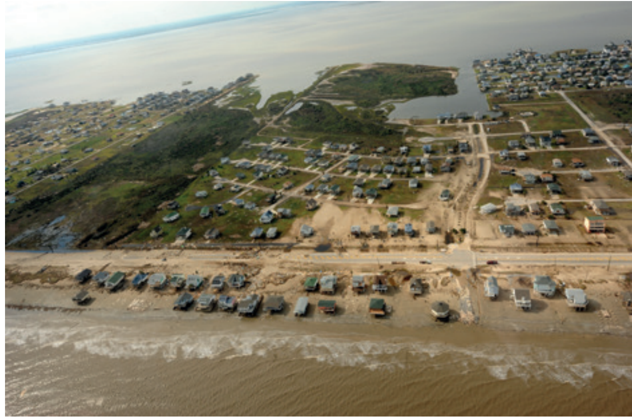
Figure 2. Galveston Island, West end, after hurricane Ike, 2008 (Photo courtesy FEMA, Jocelyn Au- gustino)
