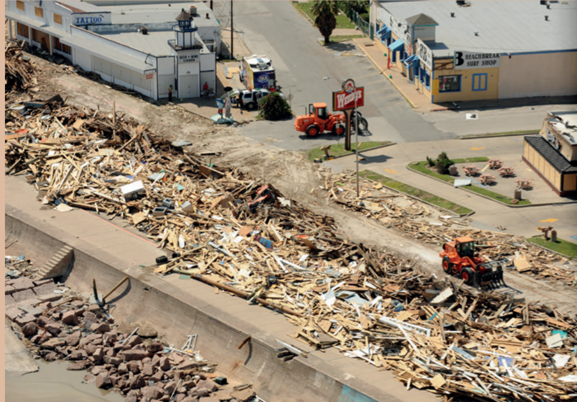
Figure 1 (below). Gathering debris on Galveston Seawall one week after hurricane Ike in September 2008 (Photo courtesy: Jocelyn Augustino, FEMA).
