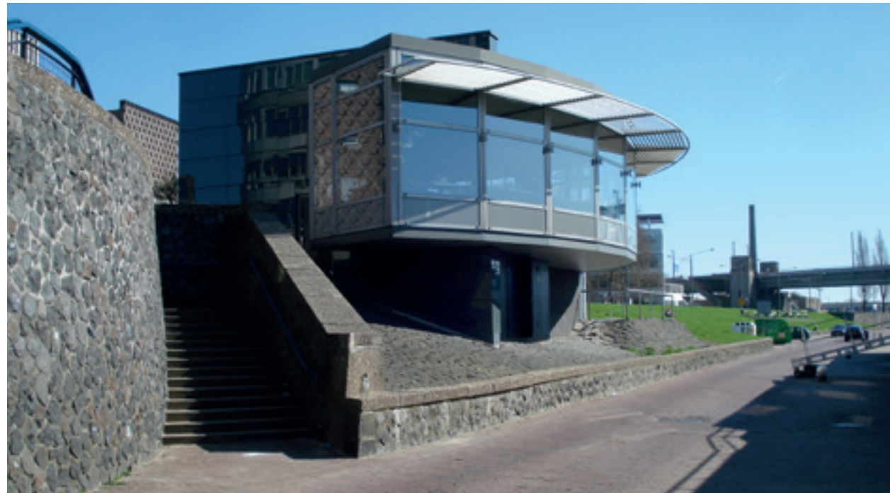
Figure 2. MFFD Arnhem, flood defense incorporating city information building (photo courtesy Mark Voorendt).
