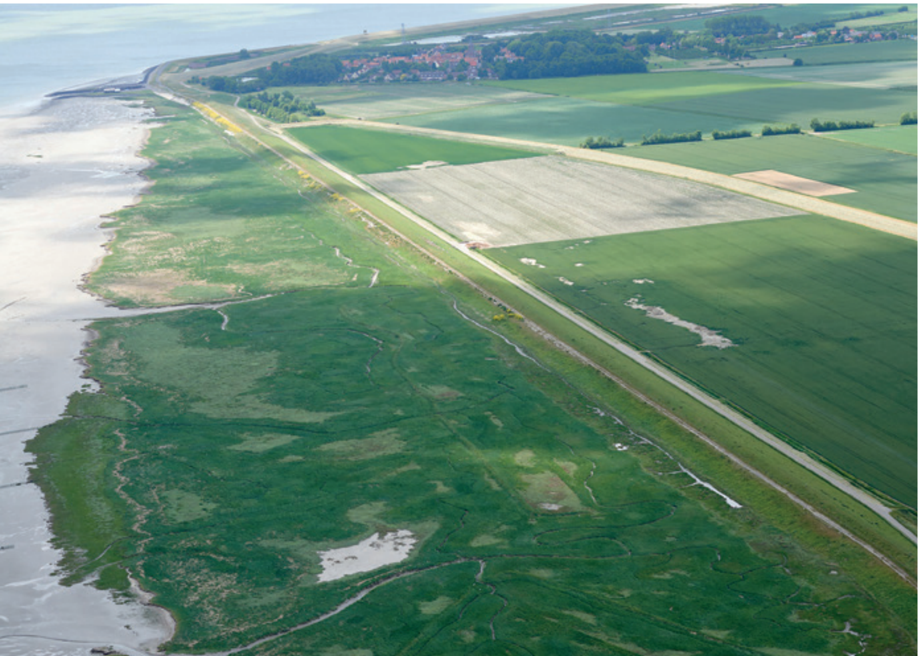
Figure 1 (below). Dike along Western Scheldt at Ellewouts- dijk with green fore- shore accomodating wave attenuating
