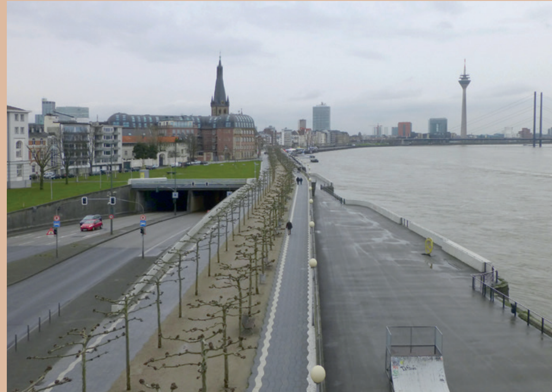
Figure 1. Multifunctional flood defense in Dusseldorf, Germany; with at the left the northern car traffic tunnel entrance and at the right the Rheinwerft quay along the river Rhine. (Photo courtesy Mark Voorendt)
