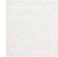
Painted original blockwork
