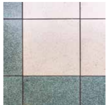
Re-used floor tiles
