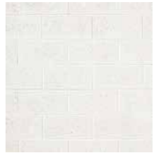
Painted original blockwork
