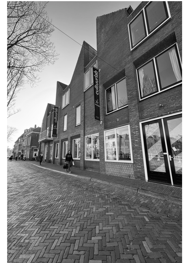
East facade of Culture lab Delft
