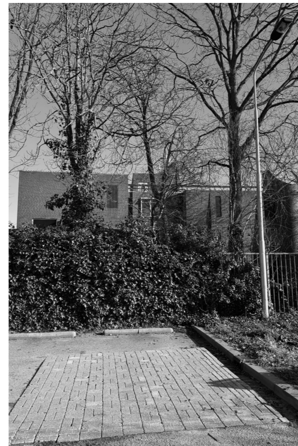
South facade of Culture lab Delft
