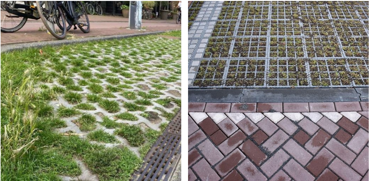
Figure 2.8: Left: Green parking using concrete pavers (Stuyver, 2021) Right: The latest development in green parking: sedum instead of grass (Bouwens, 2022)
