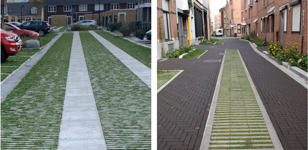
Figure 2.9: Green parking implemented in new ways (ClimateScan, 2021; SwaansInfra, n.d.)
