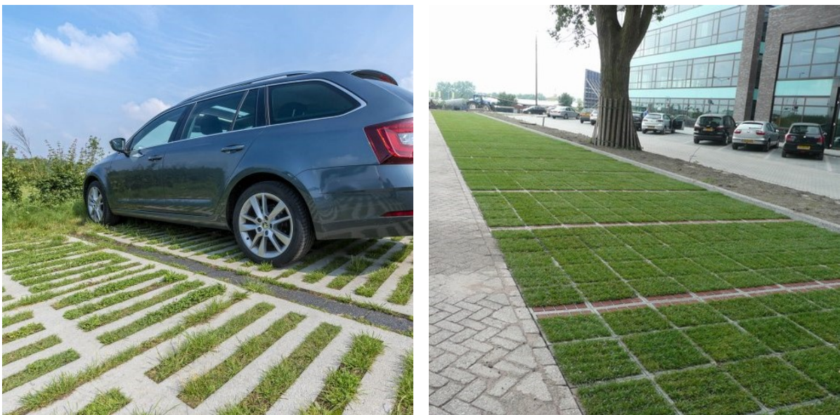
Figure 2.7: Left: Green parking using concrete tiles (Bouwens, 2022) Right: Green parking using recycled plastic (“TTE Infiltratierooster”, 2018)
