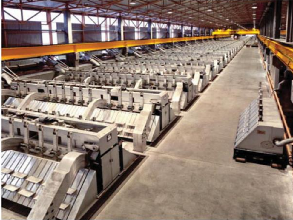
Figure 5 A modern potroom in an aluminium smelter (Kvande, 2014)
