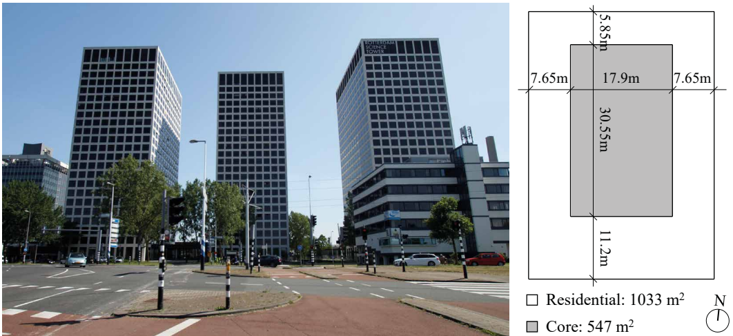
FIG. 5.2 Europoint complex in Rotterdam, the Netherlands
