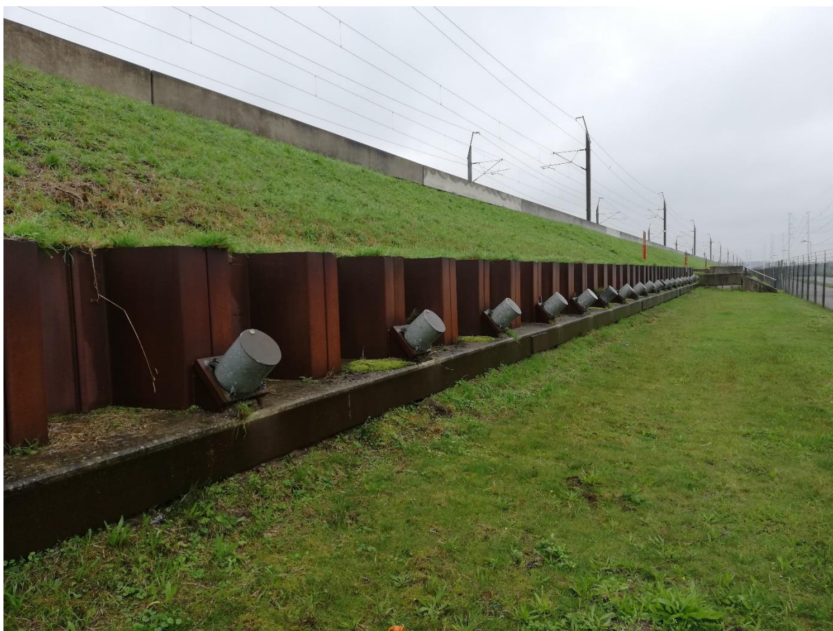
Figure 13 Post tensioned sheetpile wall
