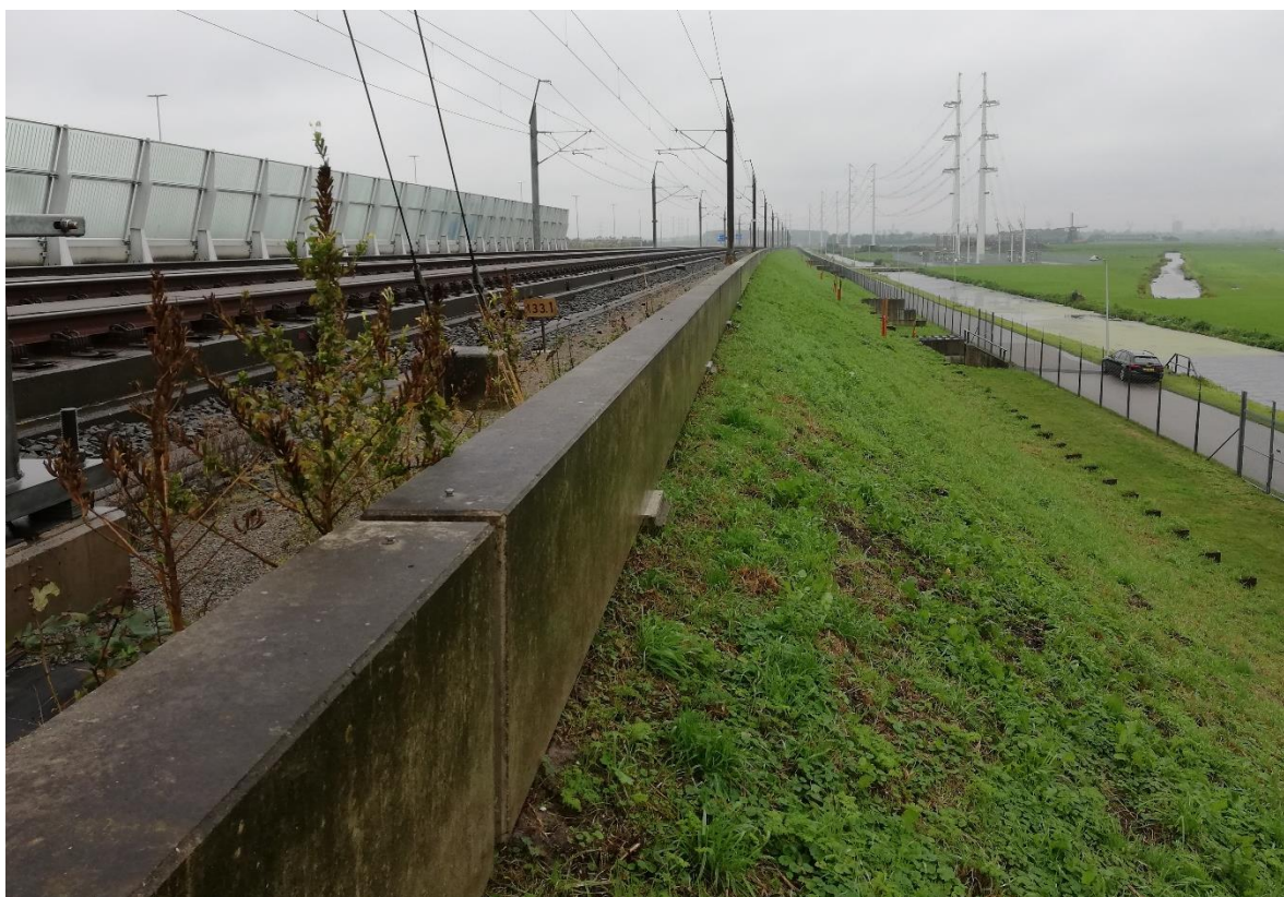
Figure 2 HSL rail structure at Rijpwetering
