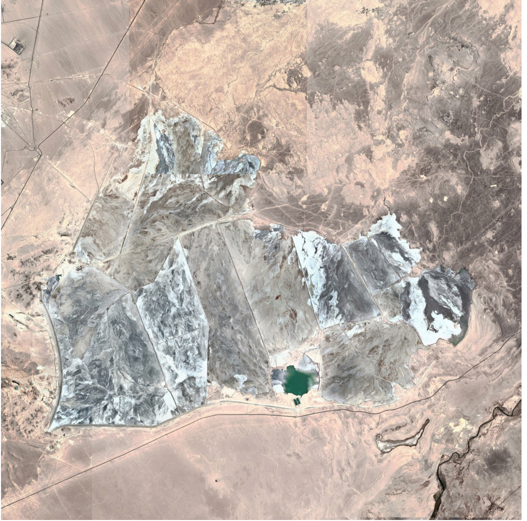
Tailing Dam Structure, Atacama Desert, Chile
