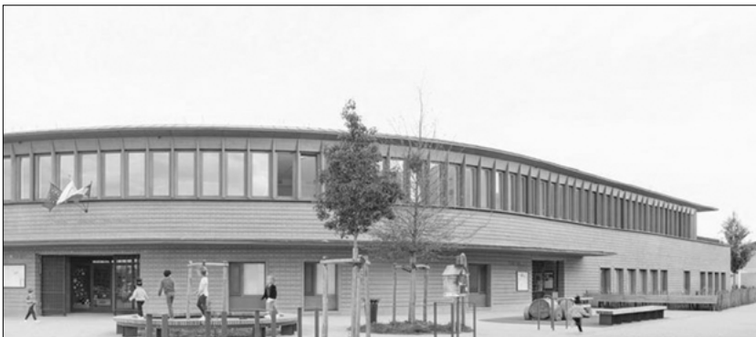
3. The Hauts du Moulin school complex in Villepreux (Yvelines), built using raw earth and timber frames.
