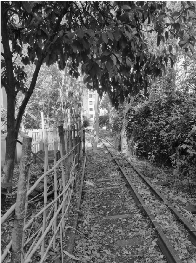
2b. Overgrowth of vegetation on an urban railway line (Qobayat-Geitaoui district)
