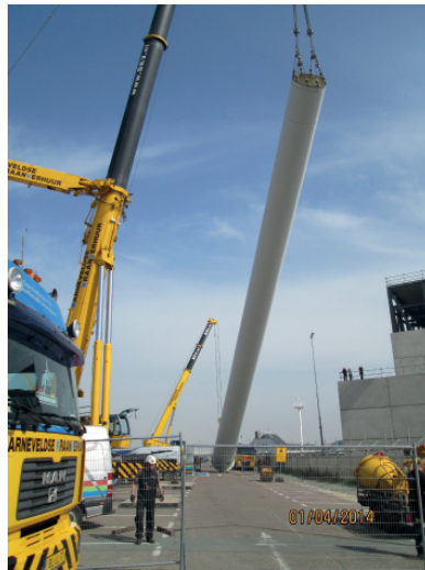
(c) Dismantling of the tower.
