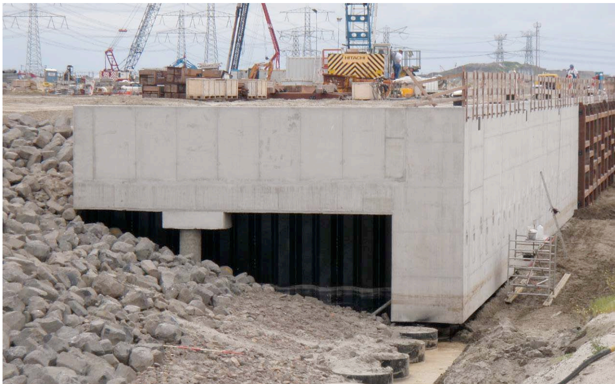
Figure 3. Eastern end of the quay wall before inundation and dredging
