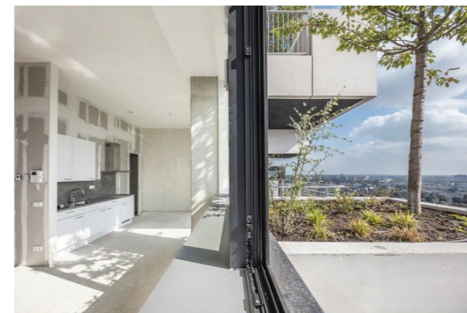
Figure 2.14: Green balcony from eye level. Can be seen it is not part of the façade itself (van Onna, n.d.)
