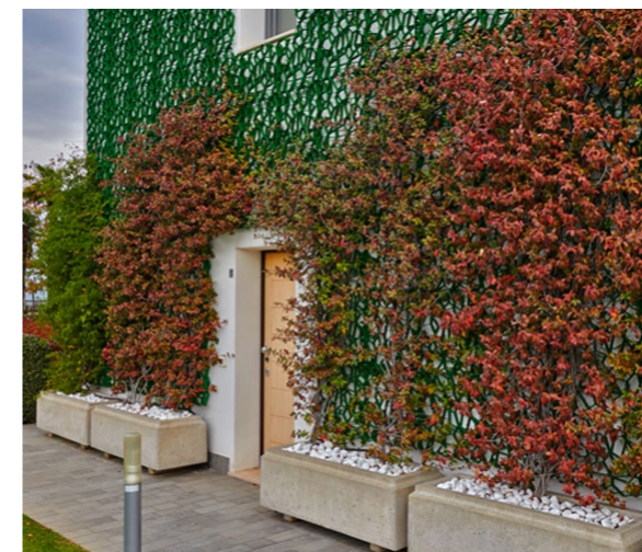
Figure 2.5: Indirect green façade rooted into concrete planter boxes at base of façade using a plastic trellis support structure (system 4) (Geoplast, 2019)
