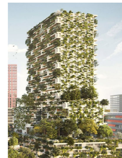
Figure 2.24: Example of a vertical forest using balconies (System 13) (Vero Digital, n.d.)
