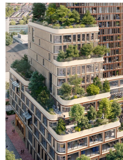
Figure 2.23: Example of a vertical forest using terraces (System 12) (Vero Digital, n.d.)
