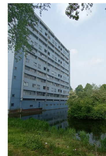
Figure 3.21: Façade surrounded by water, not easily accessible for fire fighters (Own work)
