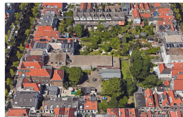
Figure 3.20: Courtyards which are not accessible by fire trucks (Google et al., n.d.)
