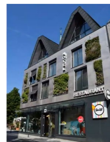
Figure 3.24: Example of VGS in patches (EFB, 2022)
