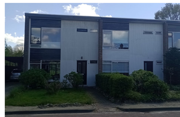
Figure 3.18: Protrusions on the façade mitigate fire spread from one house to another (Own work)
