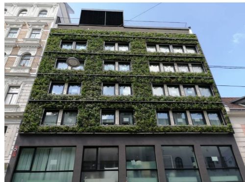
Figure 2.44: Fire breaks at every floor in a VGS on a hotel (Sempergreen, n.d.b)
