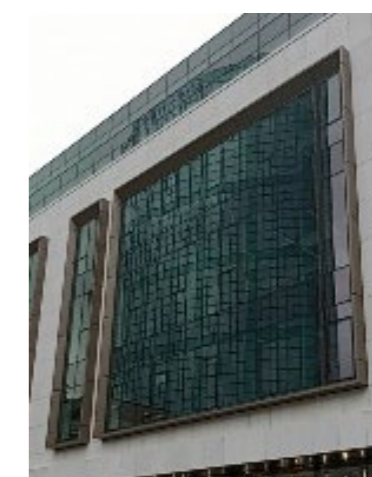
Figure 3.25: Protrusions around transparent parts (Own work)
