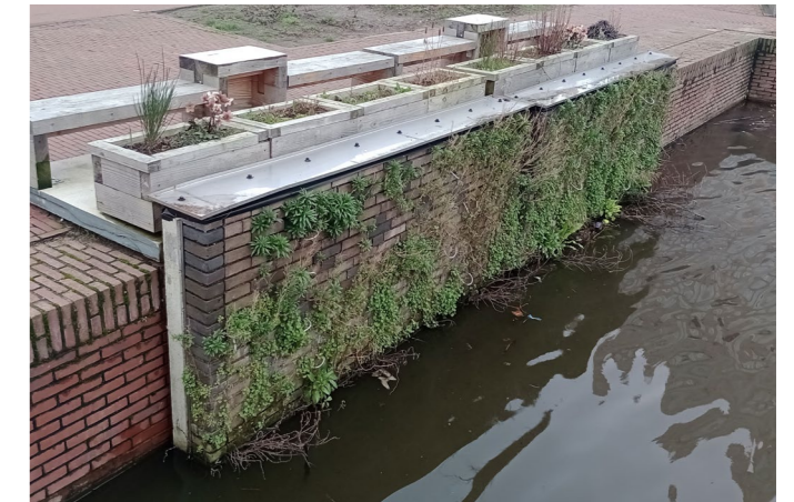
Figure 2.13: Artificial wall vegetation (system 11) (Own work)
