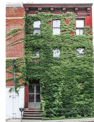
Figure 2.3: Direct green façade rooted into ground soil (system 1) (Zioandsons, 2015)
