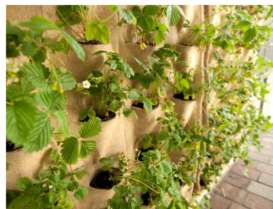
Figure 2.10: LWS based on layers of felt sheets (system 8) (Notcot, 2011)
