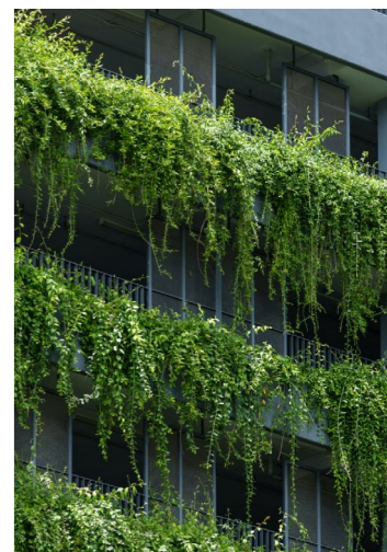
Figure 2.7: Hanging green façade rooted into pots (system 5) (Paison, 2022)
