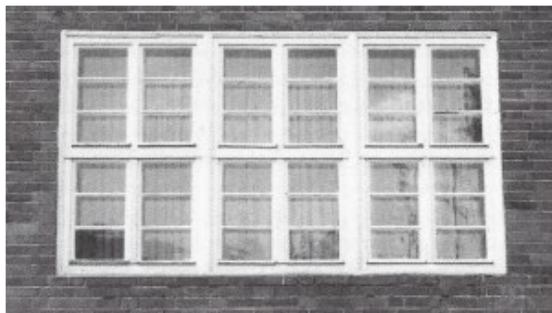
Fig. 5: Horizontality in the mullion window of the 1920s/1930s (Schrader).
