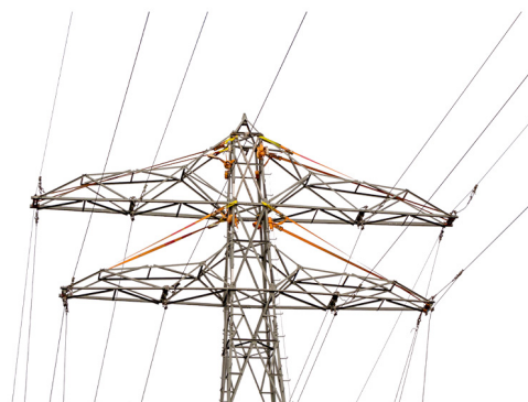
Steel frames depending on # high voltage lines demounted Rural transmission
