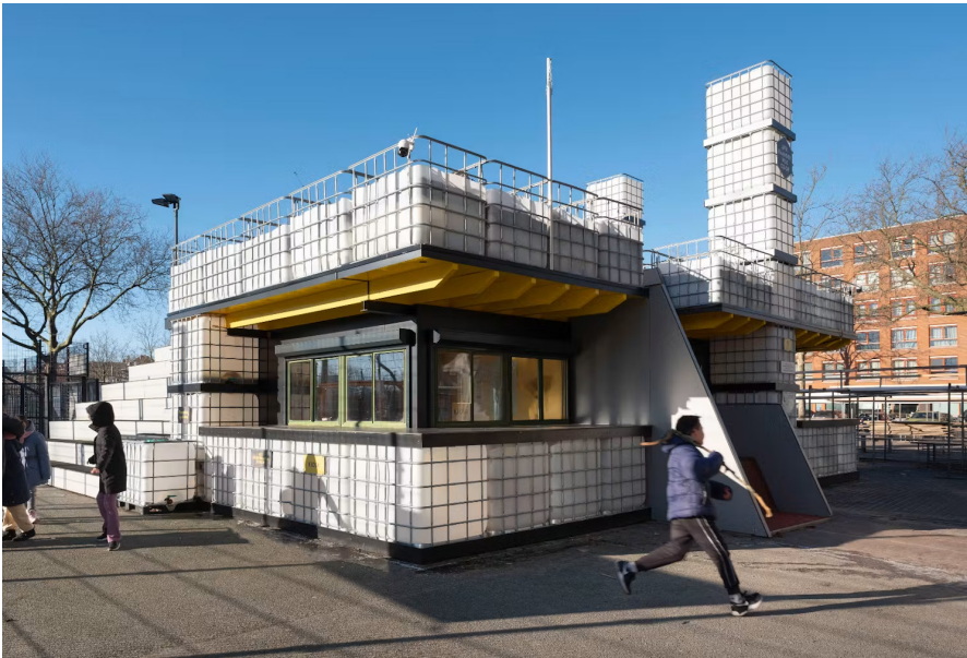
Figure 3.17 | Grondstoffenstation, Rotterdam, (Frank Gehry, 2023)
