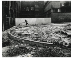
1994 Construction of treetwaling zone at Keilweg (Robert Vost)
