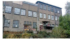
2008 Replacement of steel window frames (Stalka Groenethuis)
