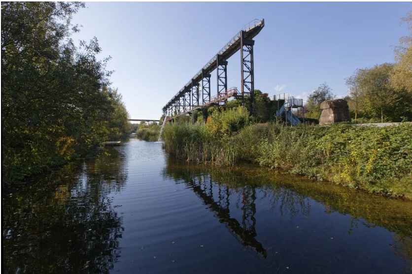
Figure 1.34 | Waterpark in Landschaftspark Duisburg. Industrial heritage transformed into a park. (Latz + Partner, 2002)
