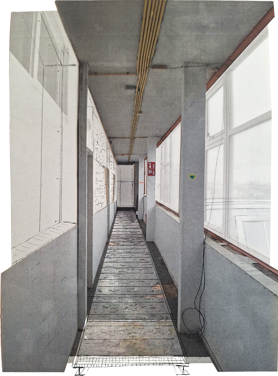
Figure 4.10 | Accessibility. Hallway with rammed demolition waste wall structure and metal mesh hallway floor.
