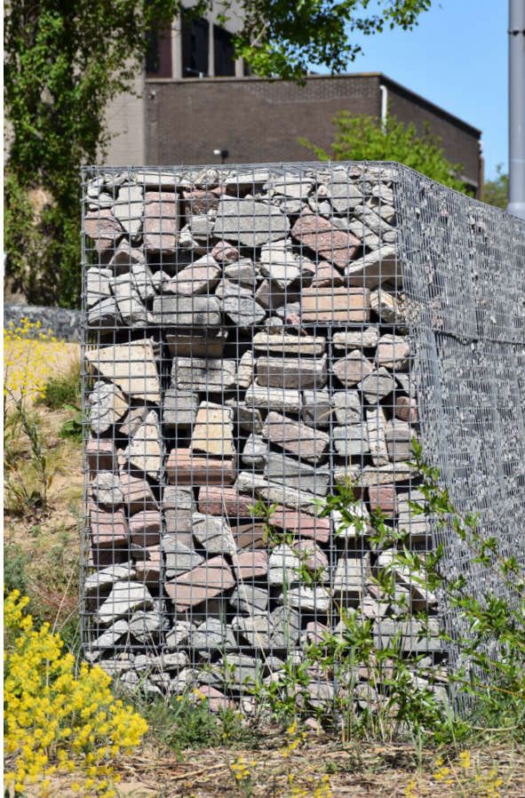
Figure 3.28 | Gabion with discarded stone. Tidal Park Keilehaven. (Floor van der Vliet, 2026)
