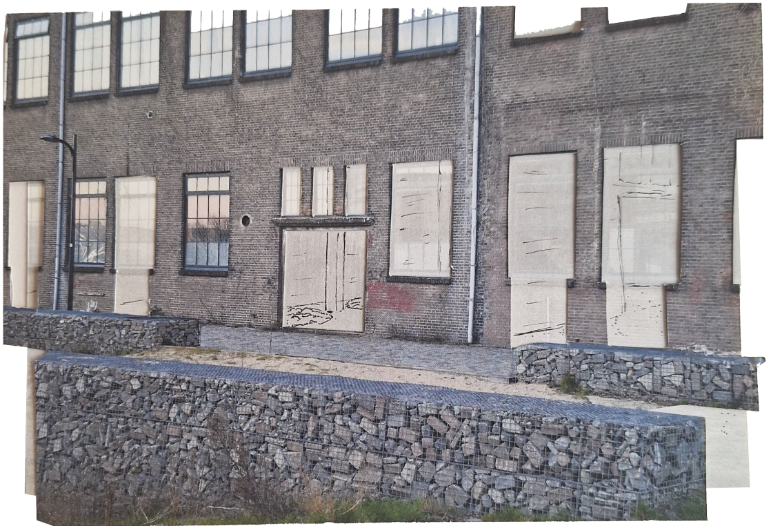
Figure 4.19 | Accessibility. Openings created in the structure increase the accessibility and porosity.
