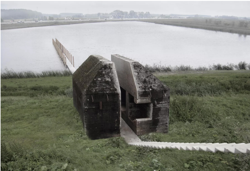
Figure 1.32 | Bunker 599. The structure was sawed open to show the interior space. (RAAAF & Allard Bovenberg, 2013)
