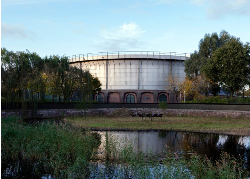
Figure 1.33 | Cultuurpark Westergasfabriek. Industrial heritage transformed into a park. (Gustafson + Porter, 2006)
