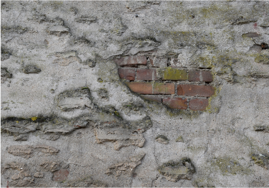
Figure 3.18 | Detail of facade of Keileweg 26-28. Layers of material and algae growth. (Floor van der Vliet, 2026)
