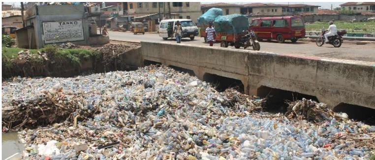
Figure 1. Plastic waste accumulation upstream of a culvert, Ghana. (Photo courtesy: TUDelft Global Initiative)
