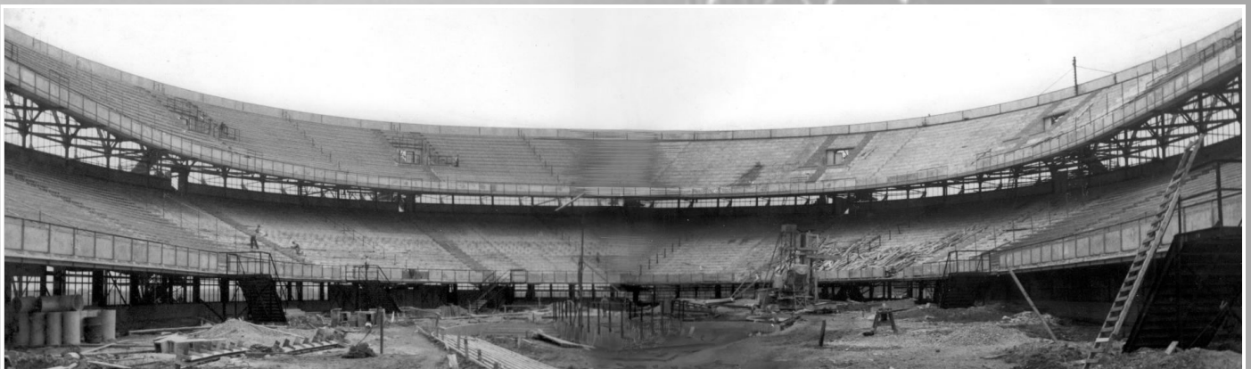
Figure 24 - Construction of the Kuip - geheugenvannederland (2010)
