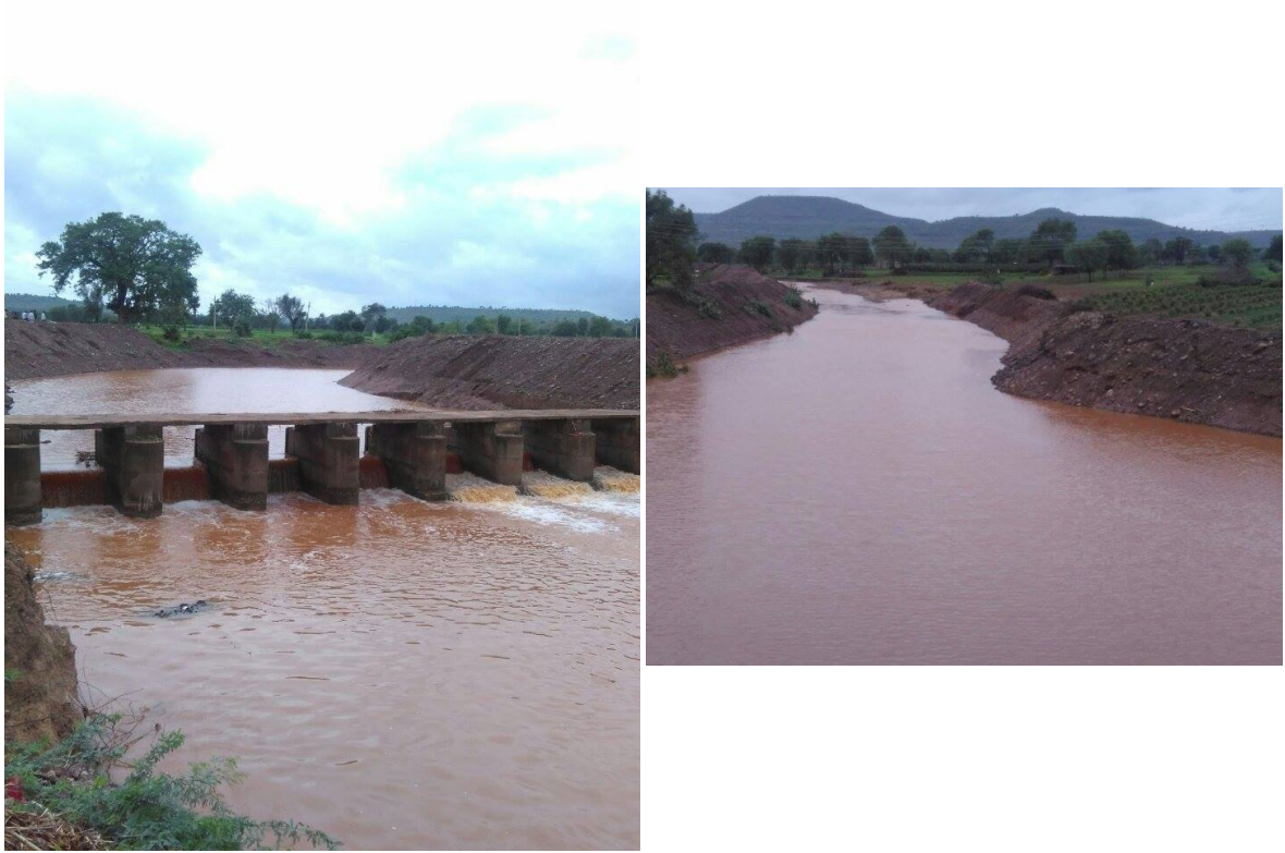
Figure E1: Pictures of some runoff interventions. Environmental flow was guaranteed, but a few changes were applied to the Dudhana River. Obstructions and deepening of the Dudhana River was realized, which resulted in significant enhancement of the water availability to local communities. Other runoff dispersion techniques also changed the situation. The pictures were taken by Prakash.
