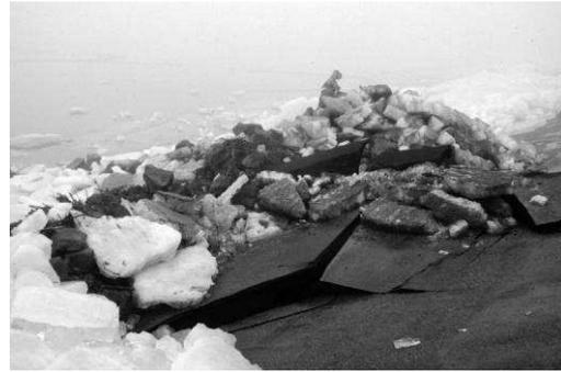
Also ships and ice forms a threat to an asphalt revetment. Fatigue is something what plays an important role in the designing and testing process of asphalt. In the Netherlands this aspect only is important when the asphalt revetment is exposed to a design storm. Under normal storm conditions there is hardly any wave attack on the asphalt revetment. After the storm the micro cracks in the layer disappear when the layer is heated up by the sun in summer time, this process is called healing.
