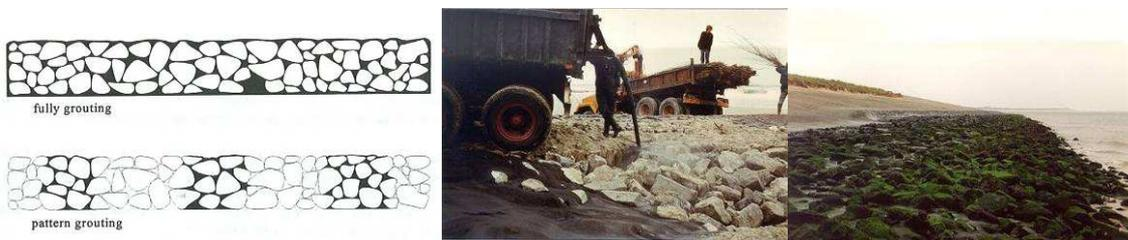
**Open stone asphalt** is mixed in two stages. First a mastic is produced which is then mixed with crushed stone (limestone 20/40 mm or 16/22 mm). A new development is that fibres are added to the mastic to increase the resistance against sagging of the mastic. A very open mixture is obtained which is water but also sand permeable. A filter construction is therefore necessary.
