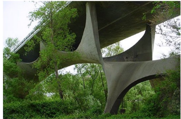
Figure 4. Basento Viaduct in Potenza, Italy, 1974 ( https://www.pinterest.com/pin/481111172670145006/ ).
