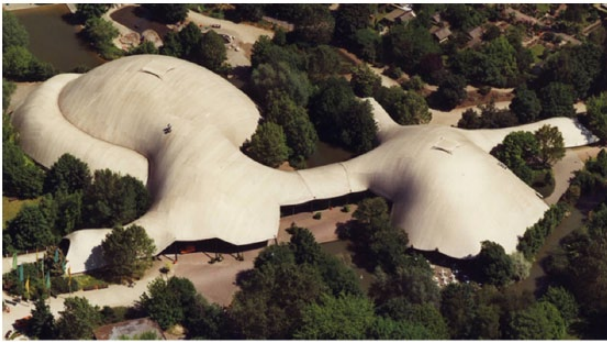
Figure 2. Roof for Multihalle in Mannheim, Germany, 1975 ( https://www.pinterest.com/pin/457045062154696404/ ).
