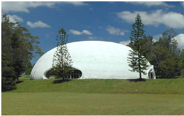
Figure 6. One Binishell in Ku-ring-gai High School ( http://www.khs82.com/dbpage.php?pg=khsphotos ).
