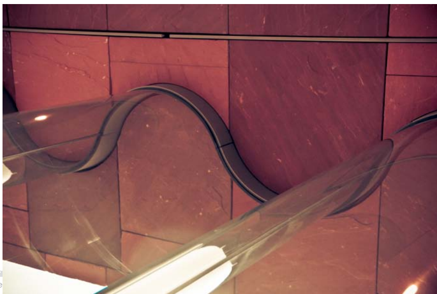
Fig.68_ View of the top detail and hidden sunscreen on the ceiling.
