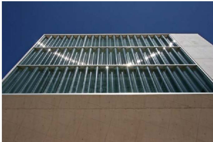
Fig.60_ Exterior view of the corrugated glass facade in Porto, Casa da Musica, OMA
