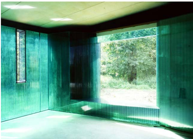
Fig.80_Interior view of the wall of the Laminata House < Glass in structures, 2003 >
