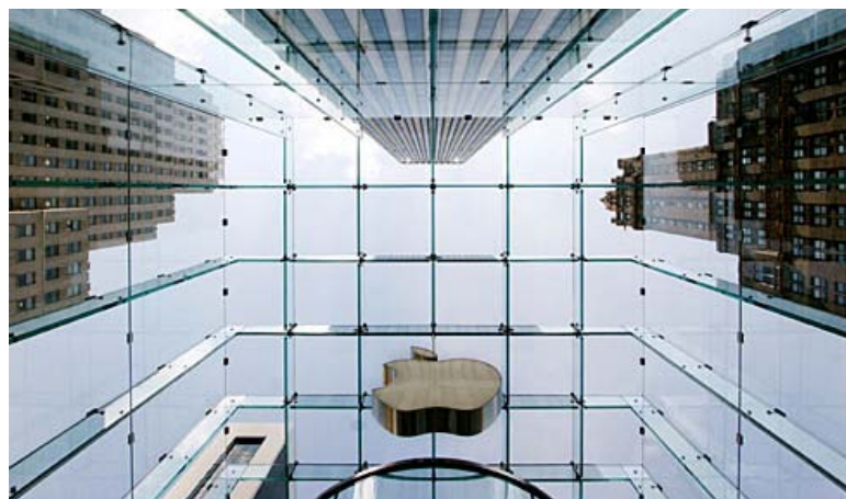
Fig.50_ View of the sky through the roof structure of the Apple cube 1.0
