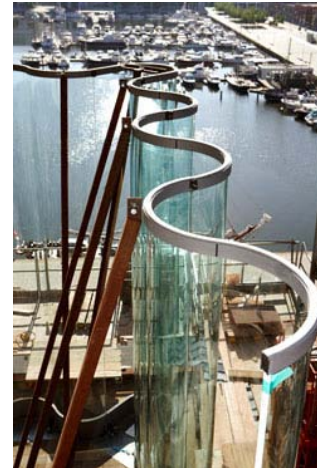
Fig.162_ Facade installation process at the Mas An de Strom. Horizontal clamping joint.
