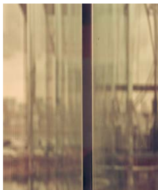
Fig.161_ Vertical silicon joint between corrugated panels in the Mas Museum in Antwerpen.
