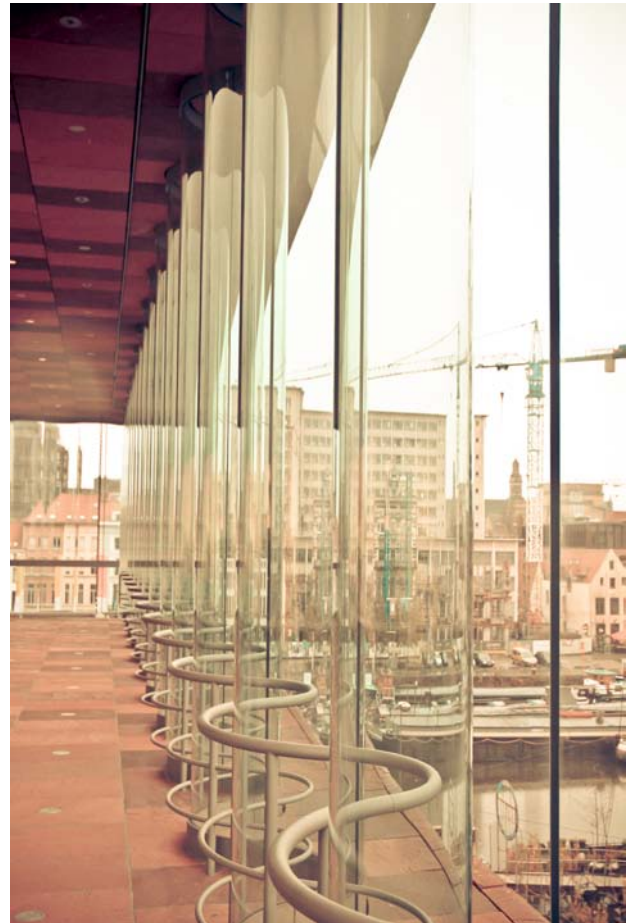
Fig.66_ Perspective of the corrugated glass facade at the Mas Museum, in Antwerp
