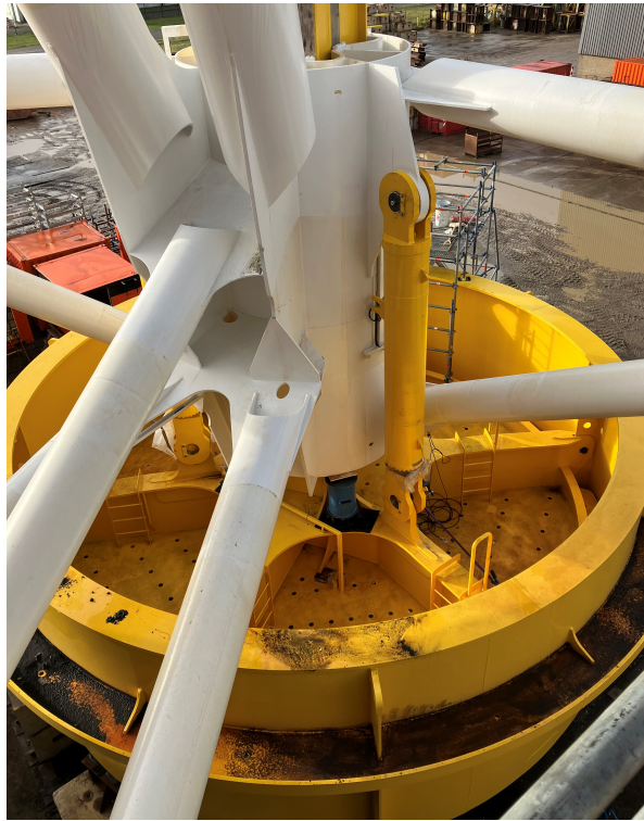
Figure 2.17: Photograph taken during fabrication of the NMS. The image shows one of the mudmats together with the upper part of its skirt.
