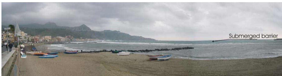
Fig. 5.12. During the first winter sea storm, waves surfing (and breaking) on the submerged barrier. Photo (9-dec-2004) of the Macine area (Giardini Bay).
