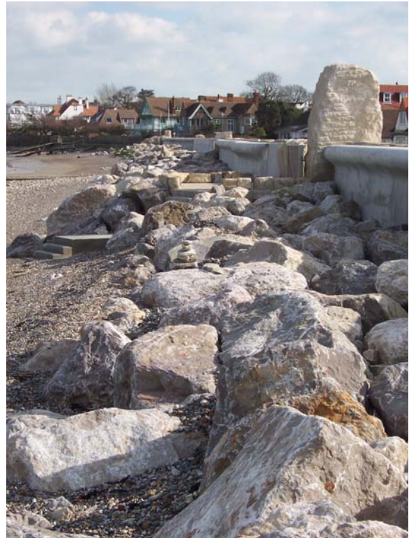
Fig. 3.56. Seaward view of the works looking towards Seaview.
