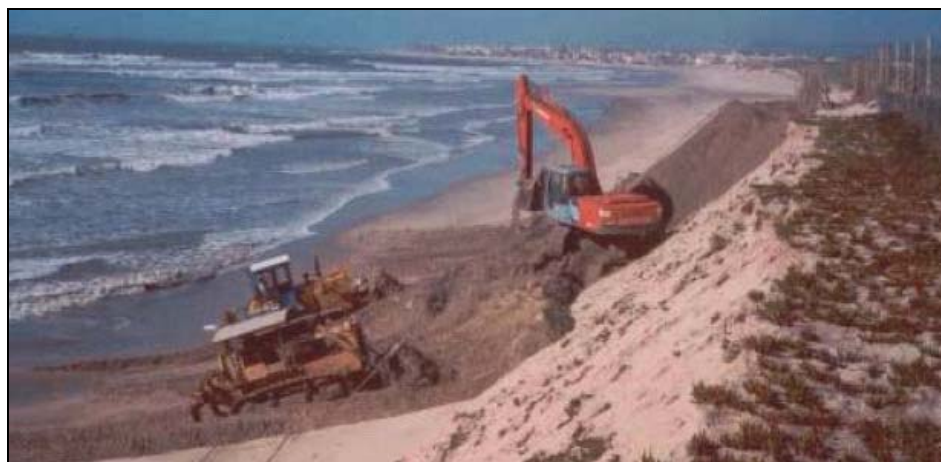
Fig. 4.64. Sand ripping works near the 5 th hole, October 2000.
