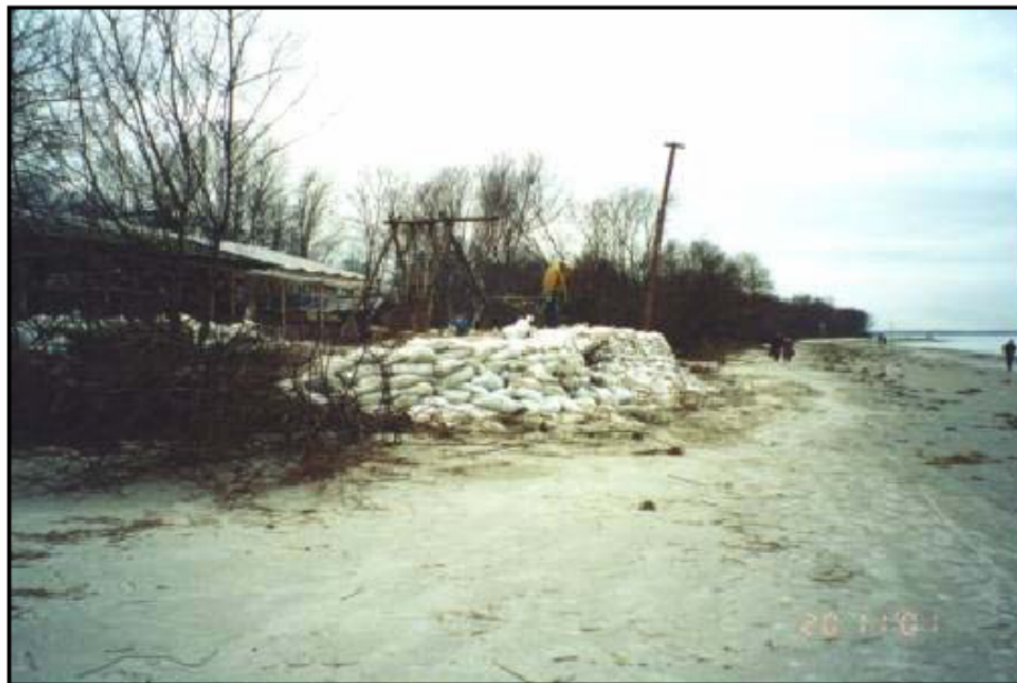
Fig. 1.42. Temporary defence measures in the place of the eroded foredune. Jurmala, November 2001
