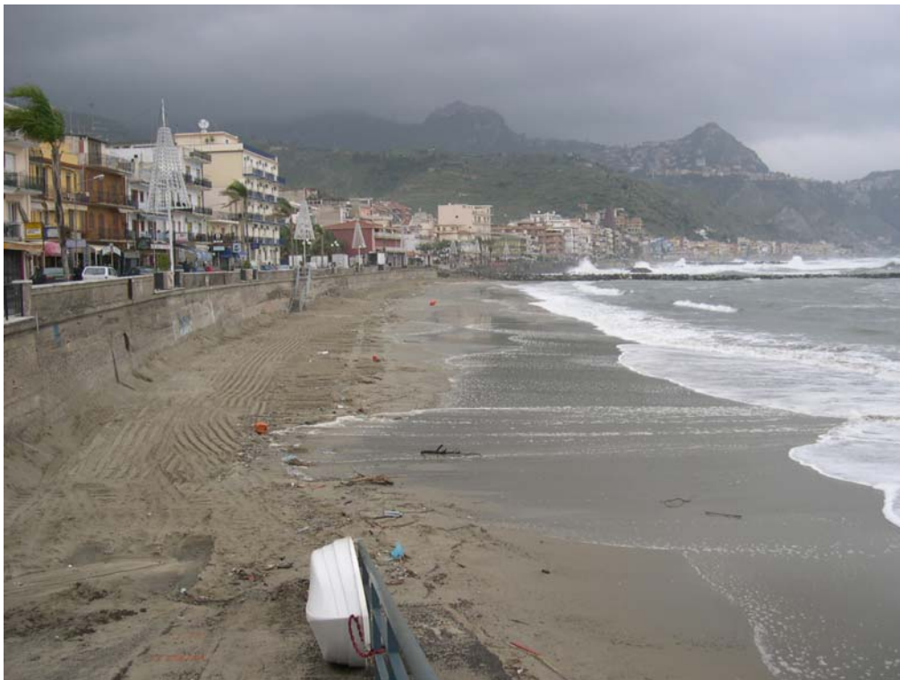
Fig. 5.9. In spite of a winter sea storm the beach is wide, and the seafront has not sustained damages. Photo (9-dec-2004) after intervention in Macine area (Giardini Bay).
