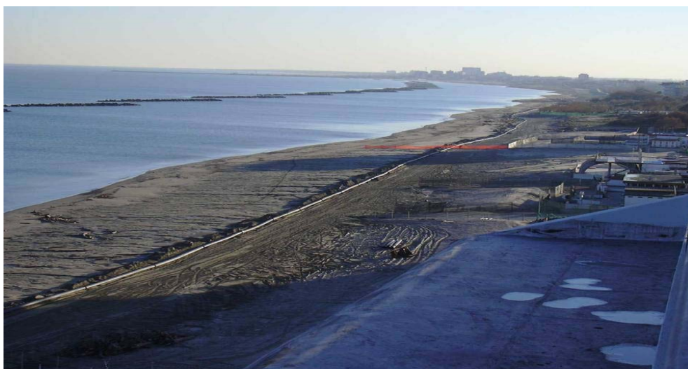
Fig.2.50. Installation of the sand-duct in Ferrara.
