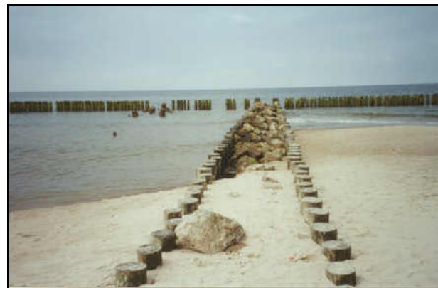
Fig. 1.9. Filling of the T – shape groyne in Dziwnow
