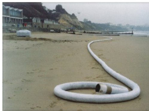
Fig. 2.45. Beach drain ready for installation
