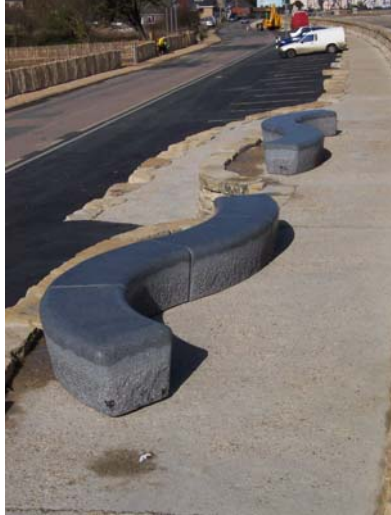
Fig. 3.58. Granite block seating on the raised footway.
