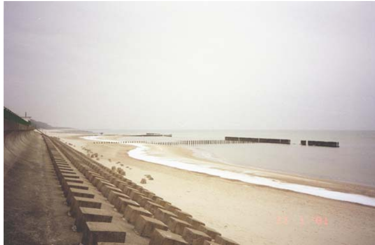
Fig. 1.25. Dziwnow: hard concrete seawall and the narrow, but existing beach in front of the seawall are visible; in the background the T-shaped groynes are visible, too
