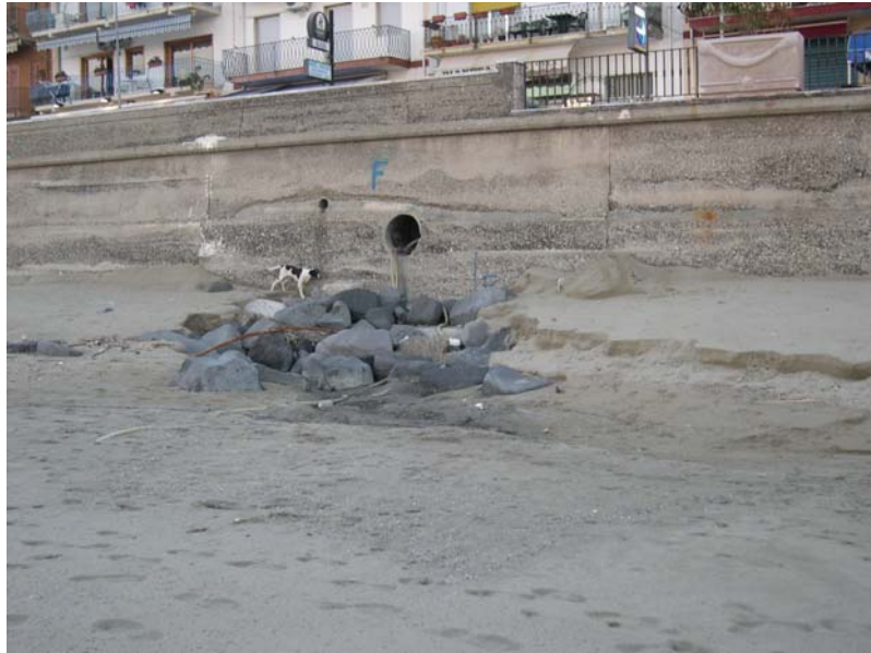
Fig. 5.7. White waste water tube.
