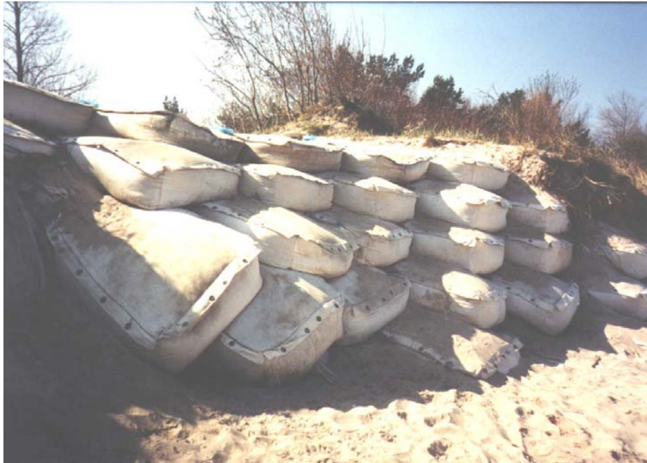
Fig. 4.69. Dziwnow: uncovered by storm event part of the artificial dune with geotextile bags core, east from hard concrete seawall
