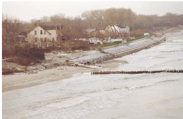
Fig. 1.24. Dziwnow: hard concrete seawall as well as rock filling seawall on the east side of hard seawall (left side of picture) are seen; on the first plan the roots of T-shaped groynes are visible; you can also see the protected property very close to the seawall.
