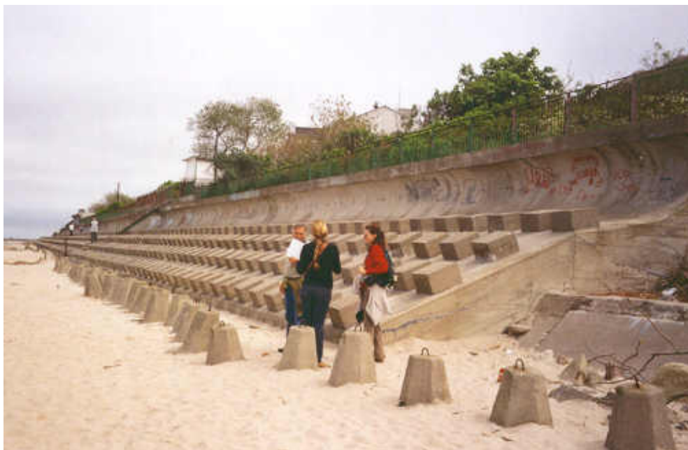
Fig. 4.70. Dziwnow: hard concrete seawall and hollow in the beach tetrapods in front of it
