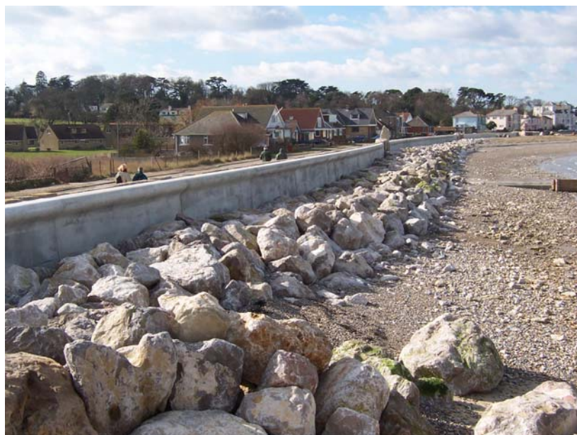
Fig. 3.57. Seaward view of the works looking towards Ryde.
