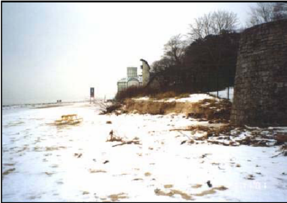
Fig. 1.43. Exposed recreation facilities after the storm surge erased the foredune. Jurmala, November 2001.
