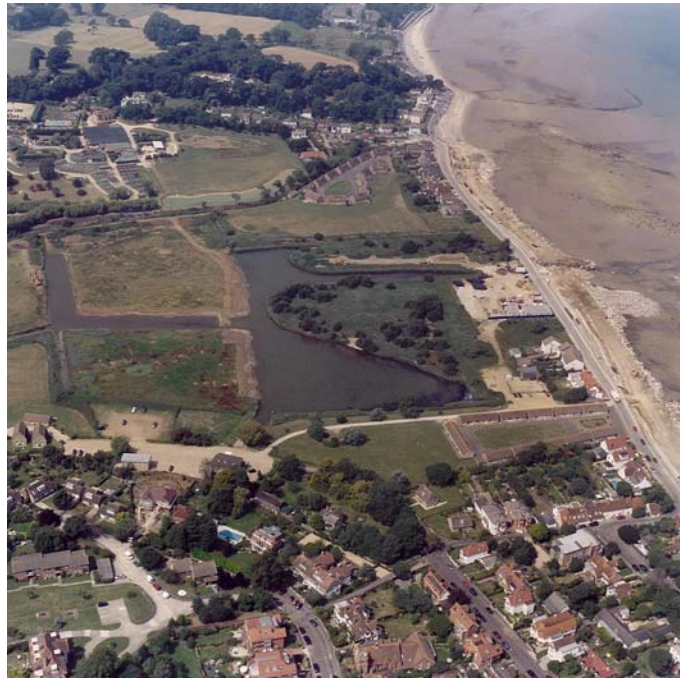
Fig. 3.53 a-b. Seaview Duver: general overview of the Duver site, showing construction work on the outfalls for Barnsley Brook watercourse.
