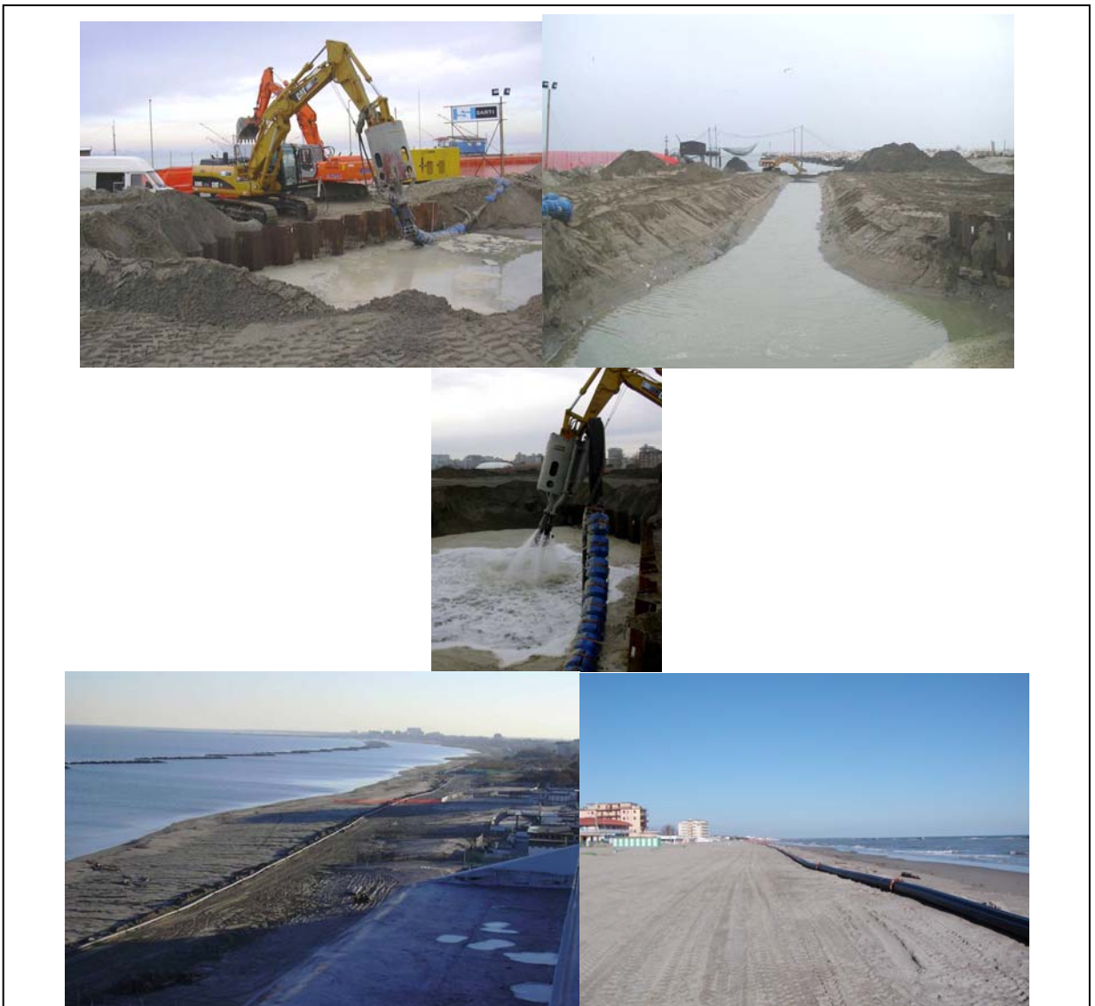
Fig. 1.38. Work in progress in Ferrara for the installation of the sand-duct.
