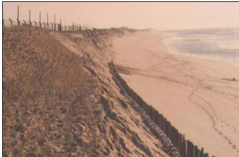
Fig. 4.63: Dune consolidation with wood piles and small sand bags, April 1999.
