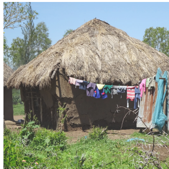
Fig. 2.7: Building type: Private house
