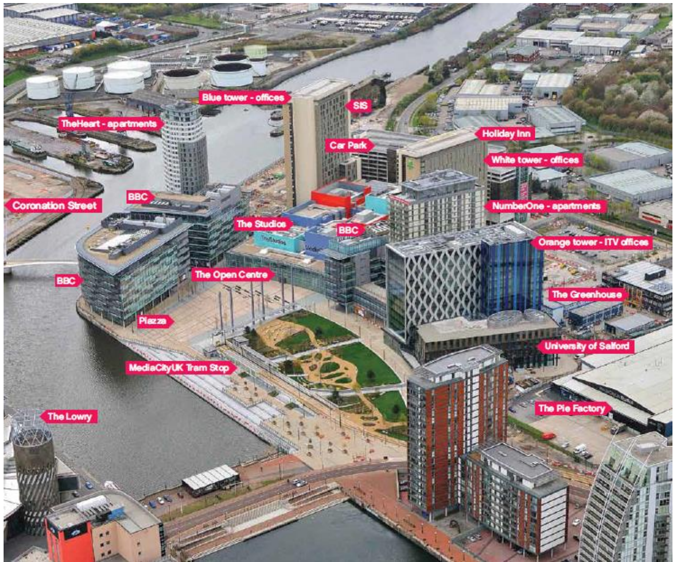
Figure 35 - Tenants and buildings in MediaCityUK (source:MediaCityUK, 2010)
