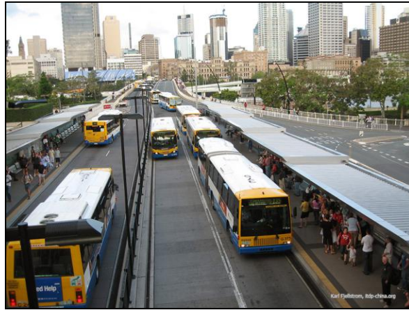
Figure 4-14: Example of passing lane in the BRT system of Brisbane. Figure reprinted from (Fjellstrom, 2007)
