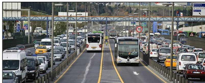
Figure 4-4: Dedicated lane in the system of Istanbul. Figure reprinted from (Talaraza, 2012)
