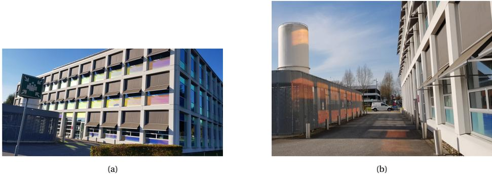
Figure 4.3: **(a)** Colored coated glass on a vertical facade of a building located in the campus of TU Delft. The color shift from window to window is very perceptible, and sometimes undesired. **(b)** The coated glass produces substantial glare, which can cause discomfort and must be avoided in critical areas where it could be a potential safety hazard.
