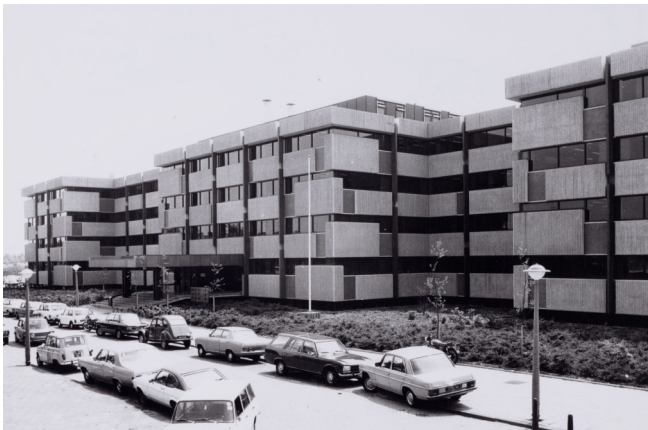
Figure 3 & 4: PI59 before and after. Source: V8 Architects
