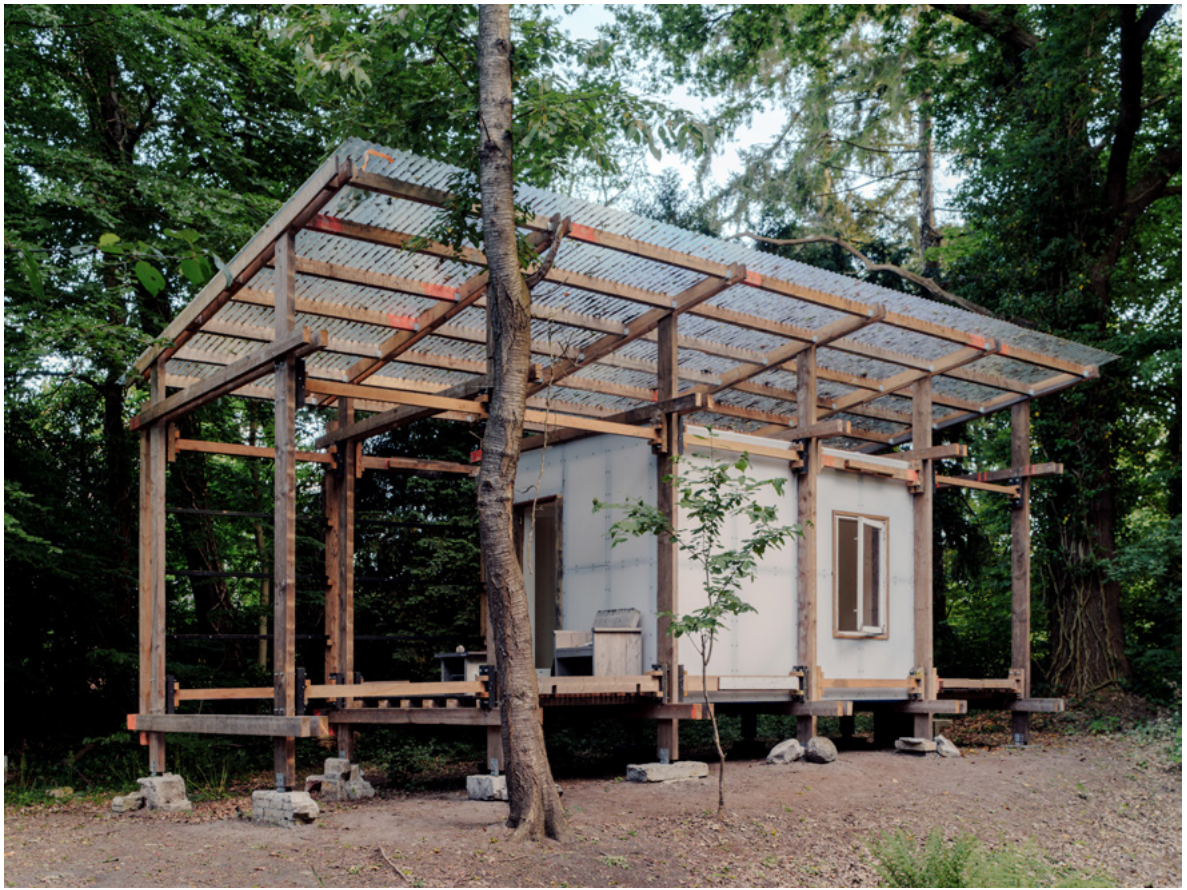
Figure 40 (above) The Reading Room in the Forest. An experimental building made almost entirely from bio-based demolition waste. Photograph by Riccardo De Vecchi.
