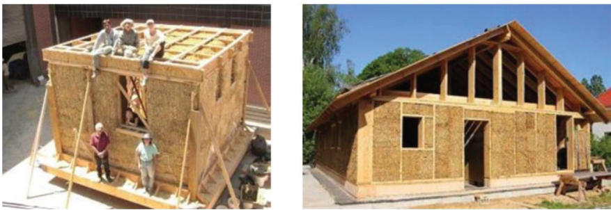
Figure 13.12 Construction of a single-storey house using straw [114].
