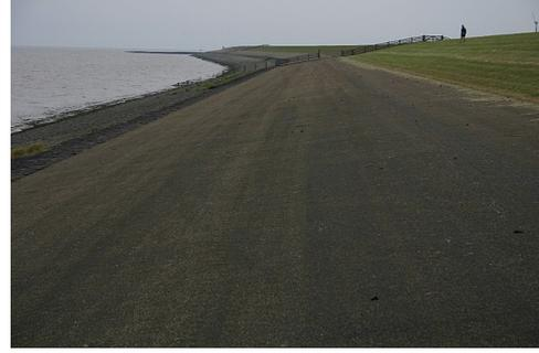
(b) Hydraulic asphalt concrete (Deltares, 2015b)
