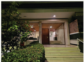
Exterior of an apartment building at the corner of Pafos 2 and Charalambos Trikoupi streets, Enkomi
