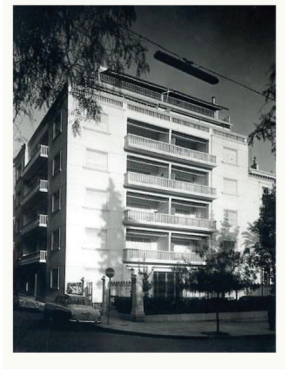
Architect: Emmanouil Loukakis. The white 11-story apartment building is a typical example of the dominant style of the 1930-1950, classifying modernism.
