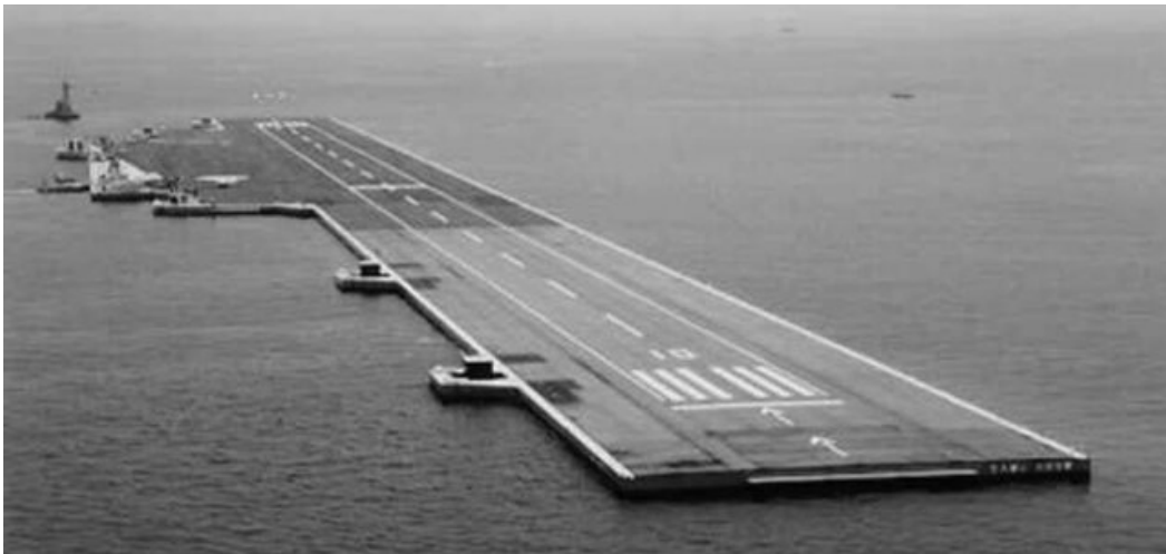
Figure 1.1: Large artificial floating island: mega-Float runway in Tokyo Bay in Japan, 1995 [7].
