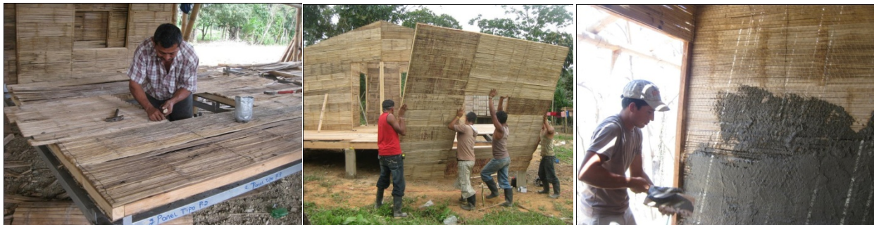
Fig. 44 Construction of esterilla panels and bamboo housing in Nicaragua (CO2 Bamboo,2010).
