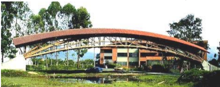
Fig.25 Bamboo bridge at technical University in Pereira (Jorg Stamm, 2010).
