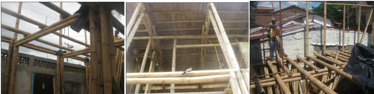
Fig. 30 CO2 bamboo renovation of house in Granada (CO2 Bamboo gallery, 2011).
