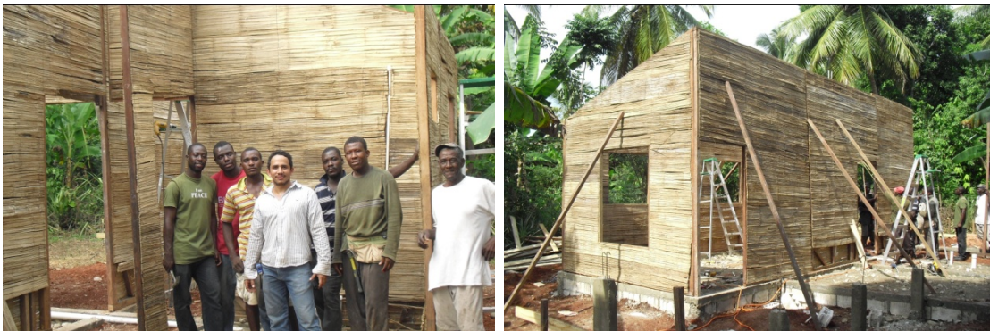
Fig. 10 First bamboo house constructed in Jacmel (CO2 Bamboo, 2011).
