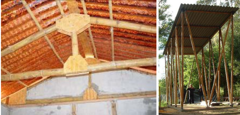
Fig. 34 Bamboo truss pilot project India (Vengala, 2002) and Koolbamboo House in Peru (Koolbamboo gallery, 2010).
