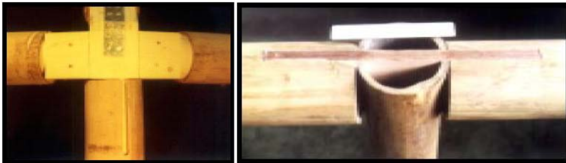
Joint designed with plywood connectors (Jannes, 2000).
