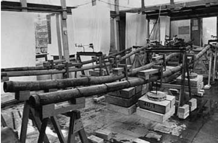
Fig. 21 Bamboo testing at Aachen University (Rottke, 2003).
