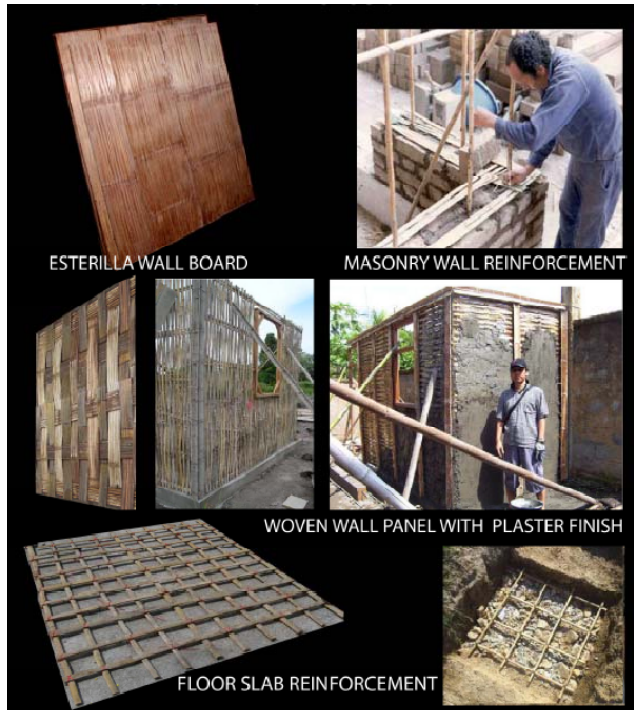
Fig. 40 Implementation of bamboo splits with low processing
