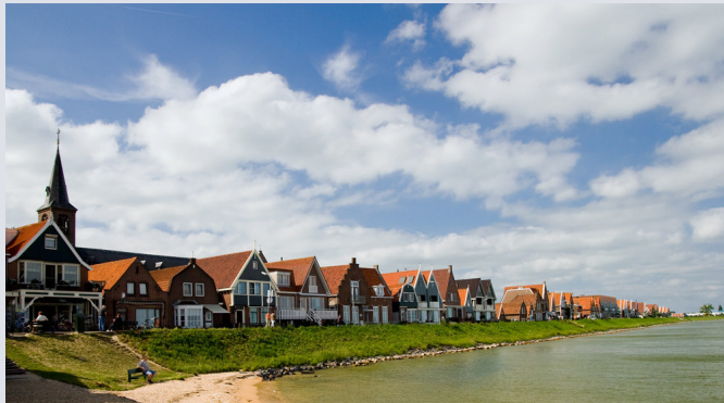
figure 18: Dike which needs to be strengthened (start-notitie)
