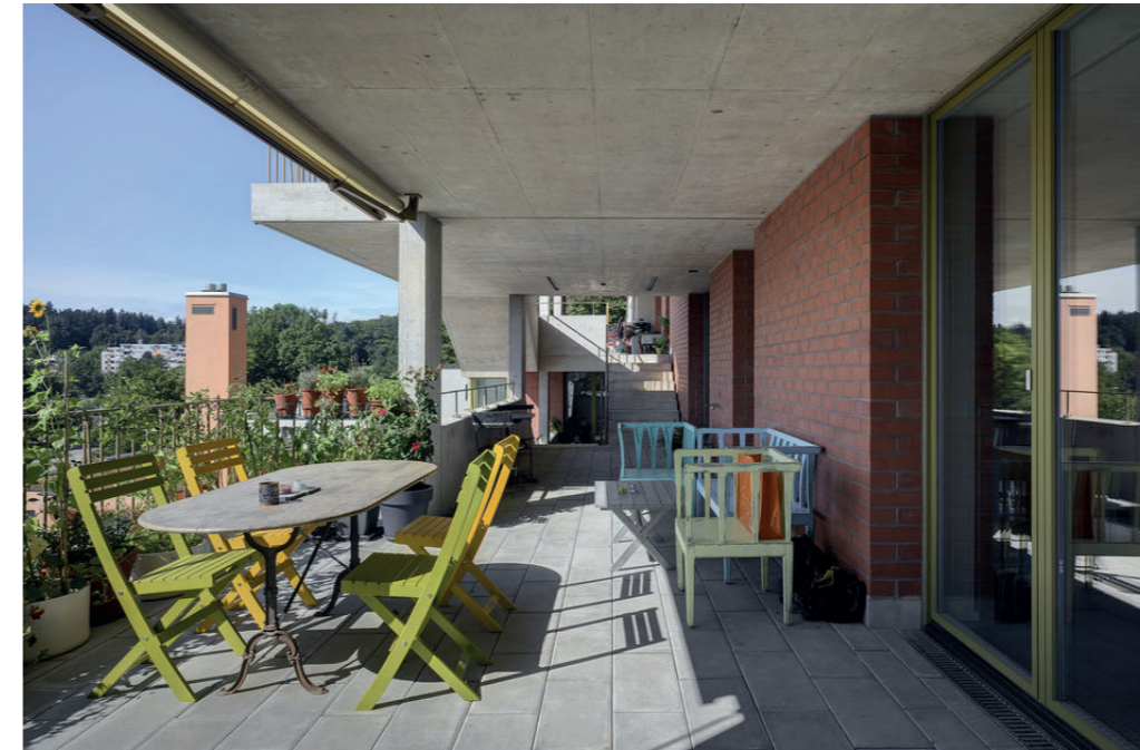
Image 35: Collective corridor with entrances
