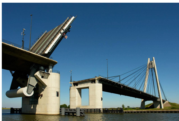
Figure 2.12: The Eiland Bridge. Retrieved from: www.heeswijk.nl
