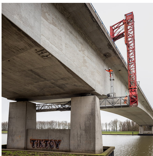
Figure 2.11: A concrete bridge during an inspection. Retrieved from: www.wagemaker.nl
