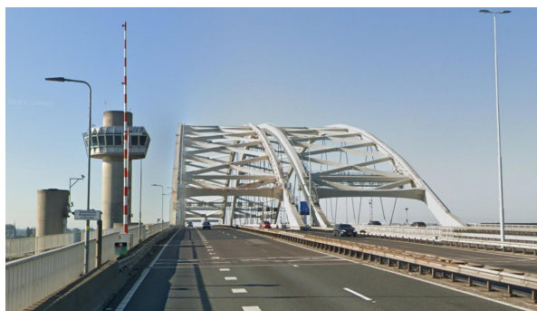
Figure 2.7: The east (left) and west (right) arches of the Van Brienoord Bridge. Retrieved from: www.capelle.ijsselektreek.nl
