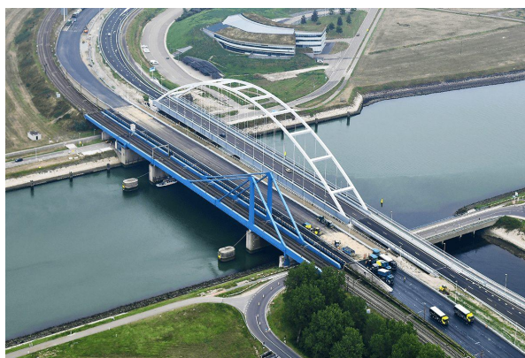
Figure 2.5: The original Suurhoff Bridge (blue) and the temporary bridge (white), installed to reduce traffic on the original structure. Retrieved from: www.hollandia.biz
