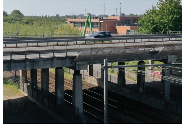
Figure 6.6: Bottom/side view of the existing Spoorweg Viaduct. Retrieved from: www.wegenwiki.nl
