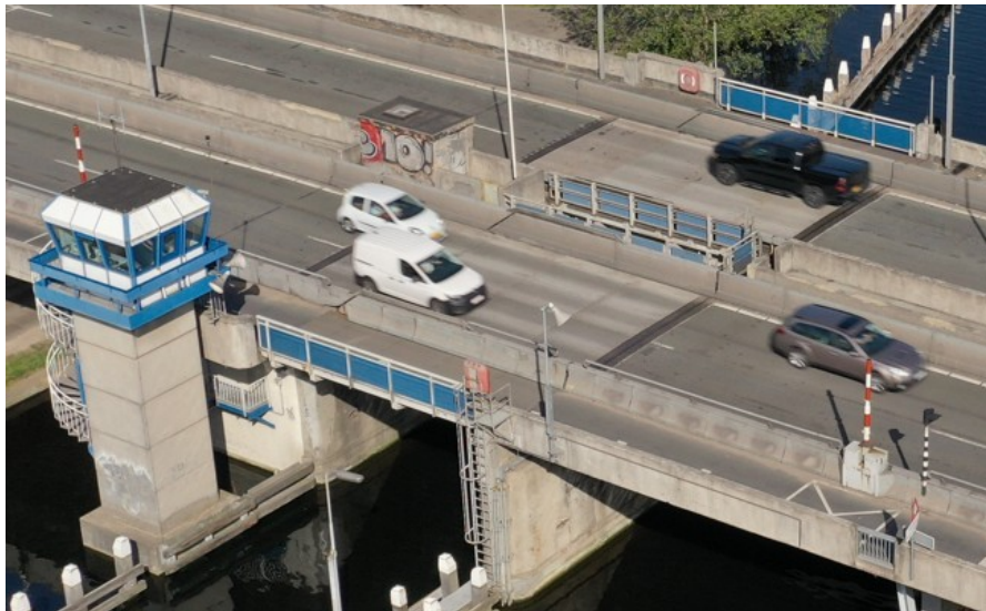
Figure 6.3: Top view of existing the Kaag Bridge, displaying the two separate bridge decks. Retrieved from: www.projecta44.nl
