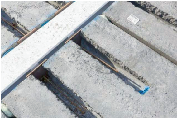
Figure 2.5 | A wet (grouted) 'demountable' connection between a hollow core slab and an integrated steel beam in the temporary Amsterdam court house (Cepezed Projects).
