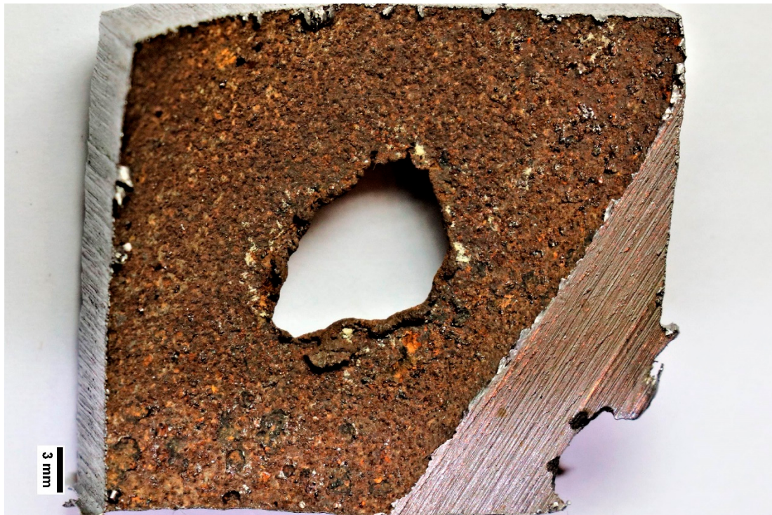
Figure 3. An inner surface of the failed elbows.
