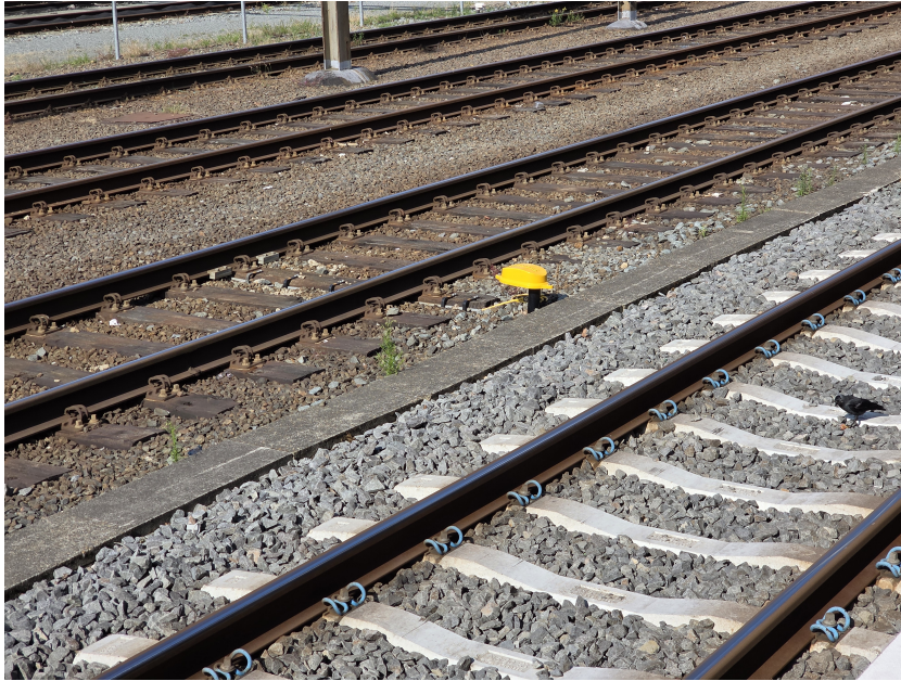
Figure 3.11: Two common forms of sleepers in the Netherlands (photo taken at Amersfoort Centraal). Flat, wooden sleepers at top of image. Sloped, concrete sleepers at bottom of image.
